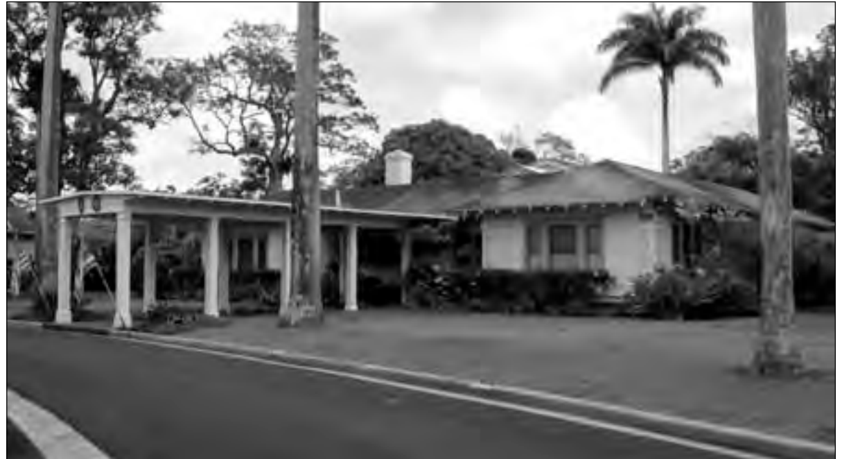
Quarters 227, Commanding Officer's House Source: Mason Architects, Inc.
