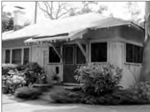
Concrete front entry steps and cheekwalls Source: Mason Architects, Inc.
