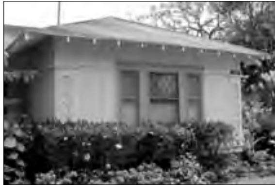
Double-hung windows at Craftsman houses Source: Mason Architects, Inc.
