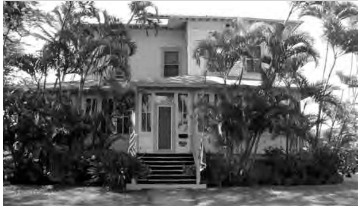
Front view of Quarters 10, Captain's Quarters Source: Mason Architects, Inc.
