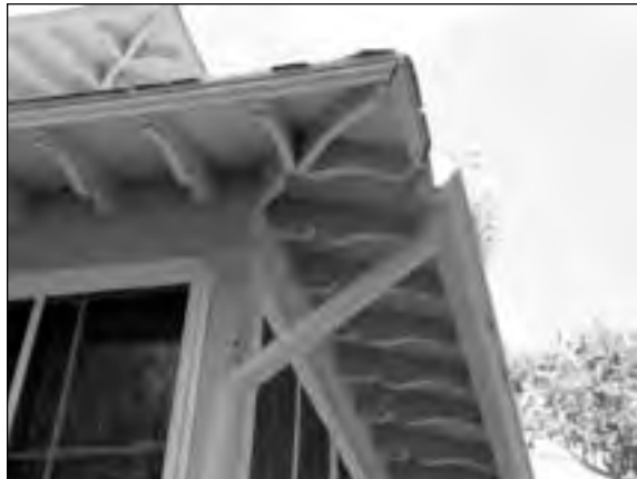
Decorative rafters Source: Mason Architects, Inc.
