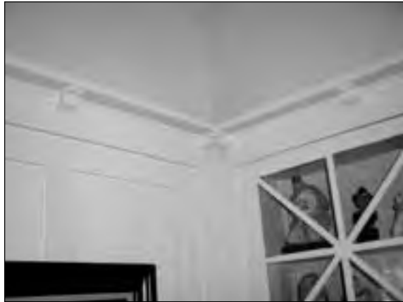
Plate rail at dining room Source: Mason Architects, Inc.
