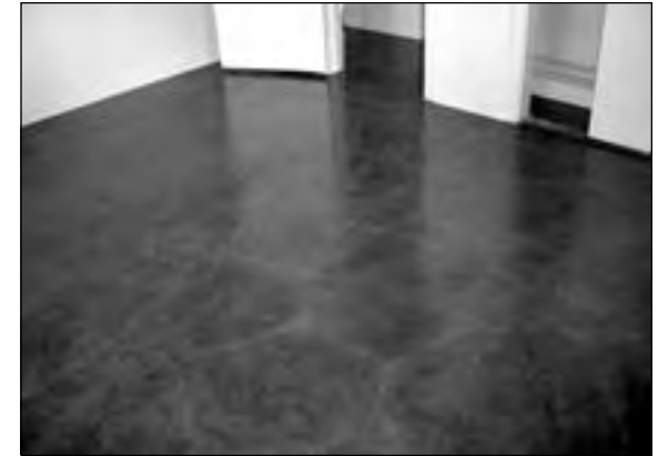
World War II unit, acid-stained concrete floor Source: Mason Architects, Inc.
