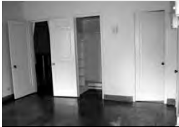
Acid-stained concrete floor and historic wood doors, Mission-style House
