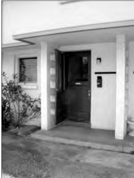
Front entry Source: Mason Architects, Inc.
