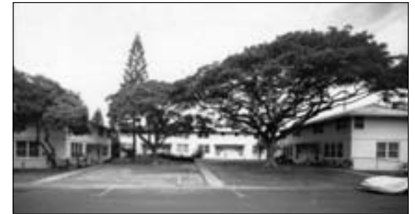
Courtyard created by three buildings in Naval Housing Area I (Hale Moku), with two-story duplexes (Facilities 176 and 178) flanking a four-plex (Facility 177) Source: David Franzen Photography
