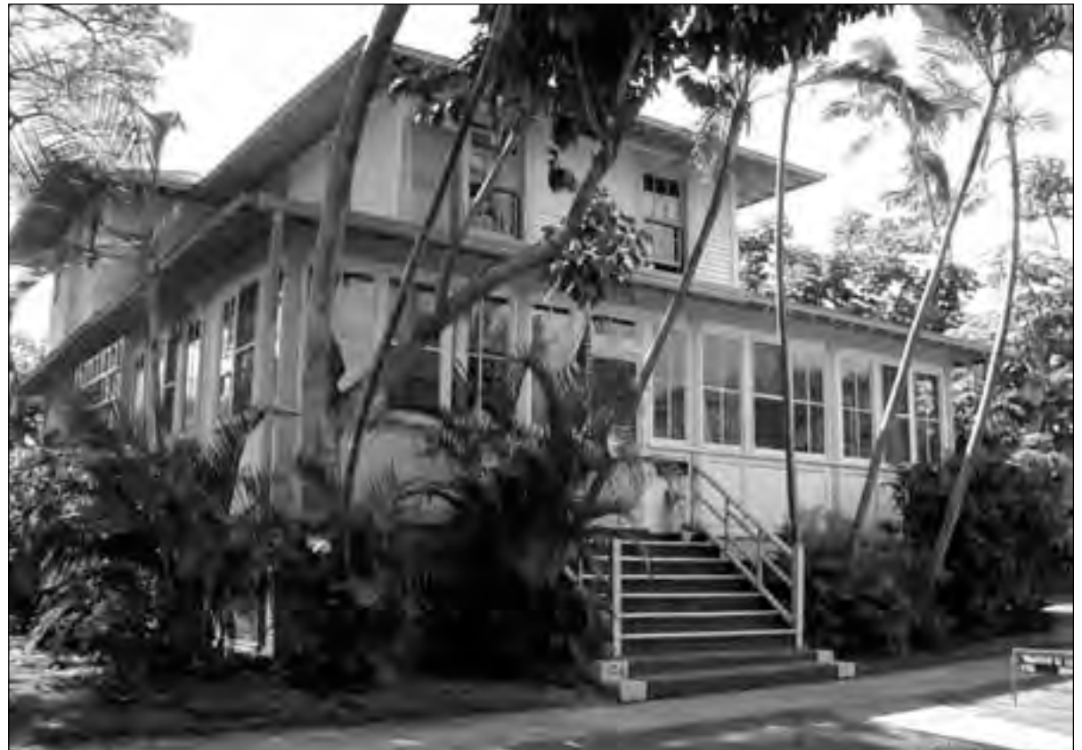
Front view of Quarters 16, NCO Quarters Source: Mason Architects, Inc.
