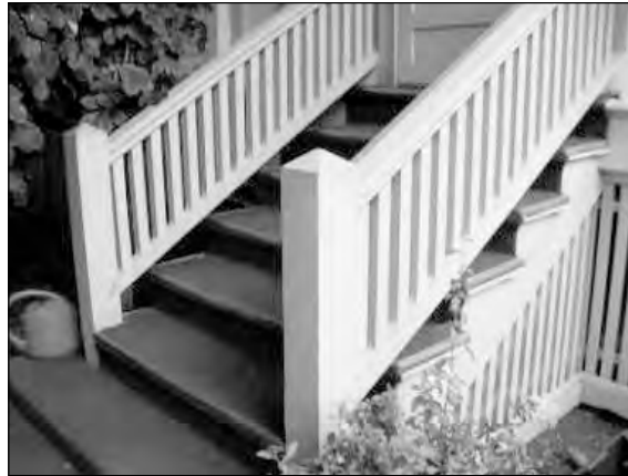
Original railing at rear lanai stairs Source: Mason Architects, Inc.
