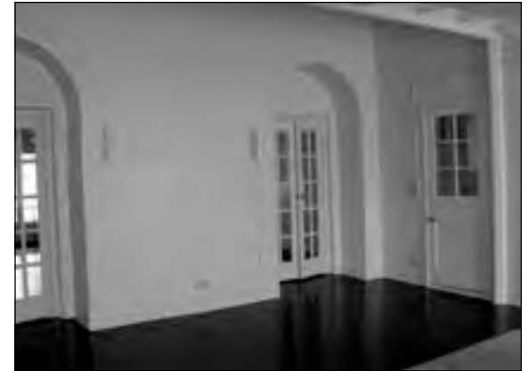
Arched doorway and historic-style door to kitchen, Mission-style House Source: Mason Architects, Inc.
