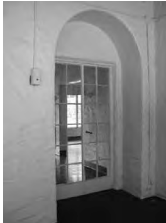
Steel doors at lanai of larger Mission-style house Source: Mason Architects, Inc.
