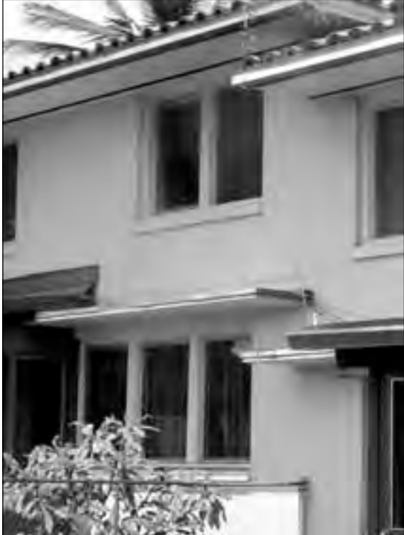
Hipped roof and flat roof over windows Source: Mason Architects, Inc.
