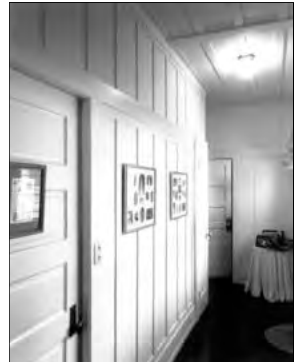
Typical interior details in Craftsman-style units Source: David Franzen Photography
