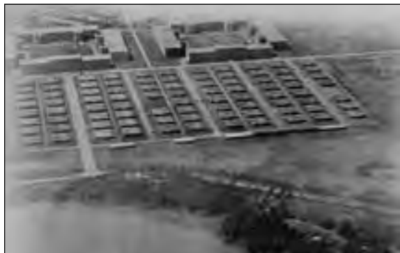
Quads and houses at Schofield Barracks Source: U.S. Army Museum of Hawaii Photo #6471
