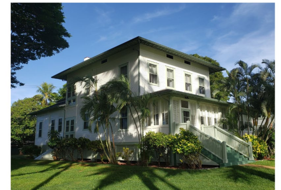
Fort Shafter, HI
