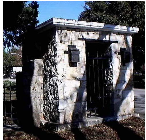
Figure 1: Camp Mabry Historic District WPA-era guard post.
