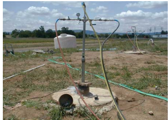
In-situ chemical oxidation using hydrogen peroxide, K-area pilot study.
