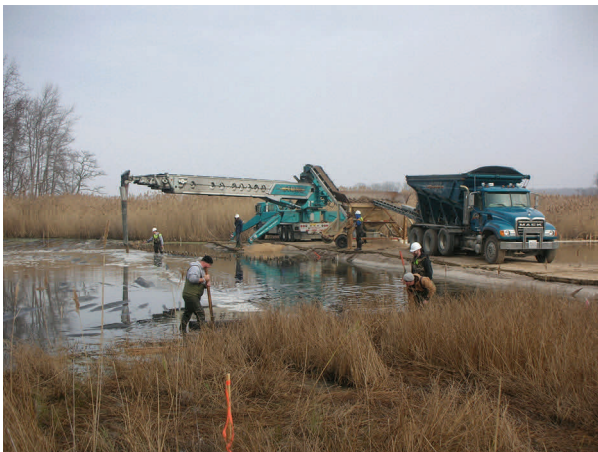
Before: A former open burning/open detonation and chemical warfare material disposal site showed signs of soil, groundwater, sediment, and surface water contamination. Personnel placed a sand/chitin mix into the pond as a sediment cover to act as a wetland buffer for plant nutrients, and to provide a food source for bacteria to break down contamination.
