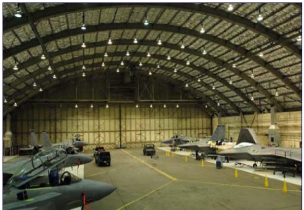
Adaptive Reuse: WWII-era hangars are currently being used for maintenance of modern fighter aircraft. This hangar supported the P-38 Lightning during WWII and Century-series fighters during the Cold War. Now it serves the nation's most modern aircraft, the F-22 Raptor.
