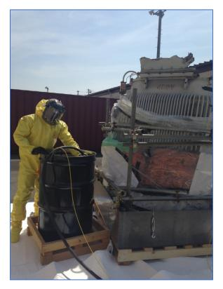
**In-house Transformer Draining** Prior to shipping contaminant-containing transformers overseas for disposal, any transformer that was leaking had to be drained. The Environmental Element was able to drain five transformers in-house, saving \$10,000 in potential contracting costs.
