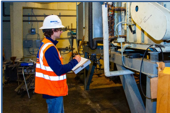
Employee conducting an asbestos inspection of piping planned for removal.
