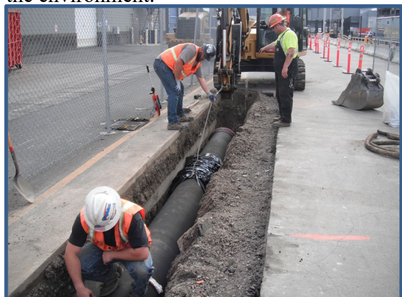
Workers replacing a 50-year sewer line along NBK Bremerton's waterfront.
