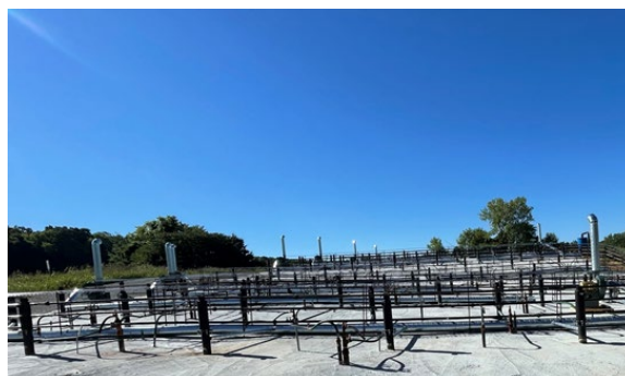
Figure 3. The innovative Area 17B insitu thermal remediation (ISTR) system will heat soil, groundwater and non-aqueous phase liquids (NAPL) within the waste pits to the boiling point of water (~100°C) for effective extraction and treatment that will optimize restoration timeframes.
