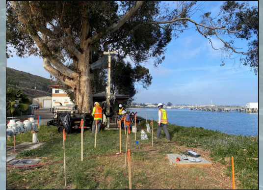
UST 105 corrective action implementation
