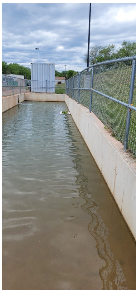
Camp Rapid wash rack sediment retention pond. Pond reuses water for washing vehicles. Algae and mosquitoes would be an issue and the addition of some floating plants, an aerator, and local minnow species keeps the use of chemicals to zero.
