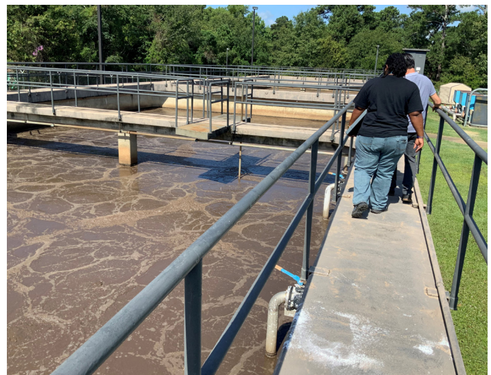
Shaw AFB Plant Operator Mr. Tony Quercero and South Carolina Department of Health and Environmental Control Inspector Ms. Shemeka Galloway review the aerator basins at Shaw AFB's WWTP.
