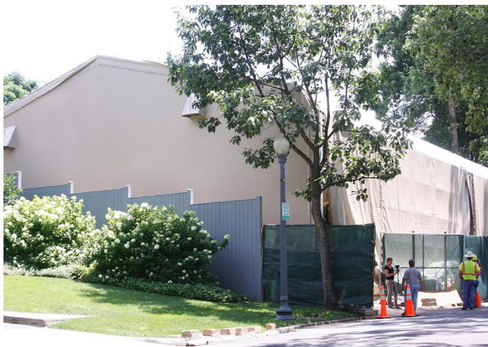
During the height of remedial efforts, a tent covered the Glenbrook Road Remedial Action site. The tent allowed the team to work safely and efficiently while they excavated and removed hazardous materials and contaminated soil.
