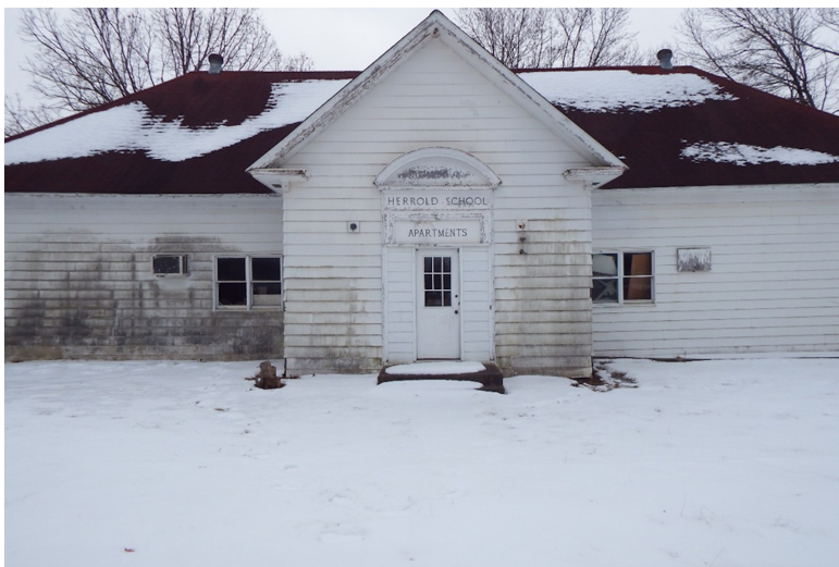
Herrold Schoolhouse, in the process of restoration to restore historical features of significance.
