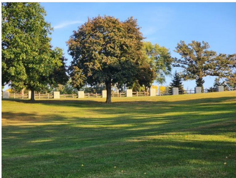
Camp Dodge's perimeter fence features 99 limestone pillars. Preservation of this unique feature involved meticulous handwork to restore the masonry.
