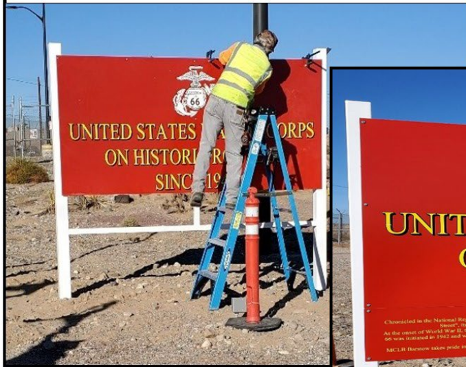
Marquee outside of Back Gate being installed
