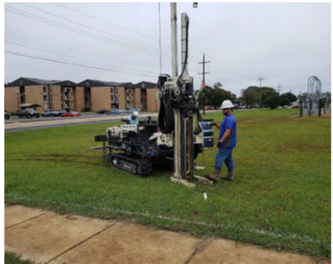
CCBldg 1725 Soil boring installation using Direct Pushing Technology (DPT) rig.
