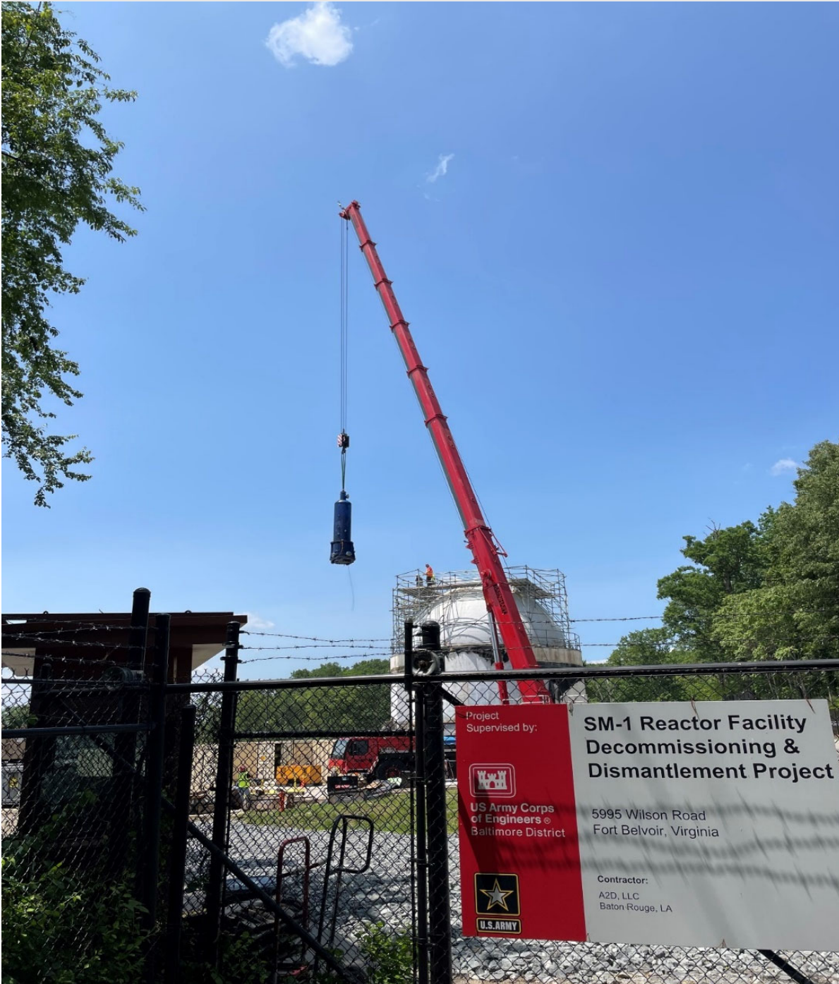
Removal of one of the reactor components – the steam generator, from the Vapor Containment Structure which housed the primary reactor systems for the SM-1 Nuclear Power Plant. The steam generator was safely removed in June 2023
