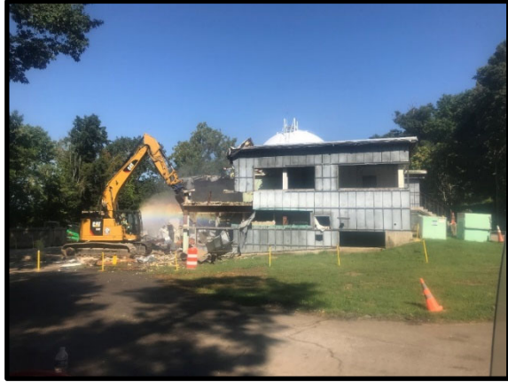
Demolition of the support building for the SM-1 Nuclear Reactor – July 2022
