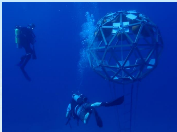
Figure 8. Engineer divers provided by the Navy installing coral “arks” supporting NIWC, Harvard, and San Diego State coral mitigation study.
