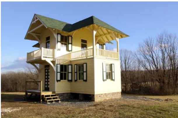
THE RESTORED RANGE HOUSE AT FORT INDIANTOWN GAP, PENNSYLVANIA.
