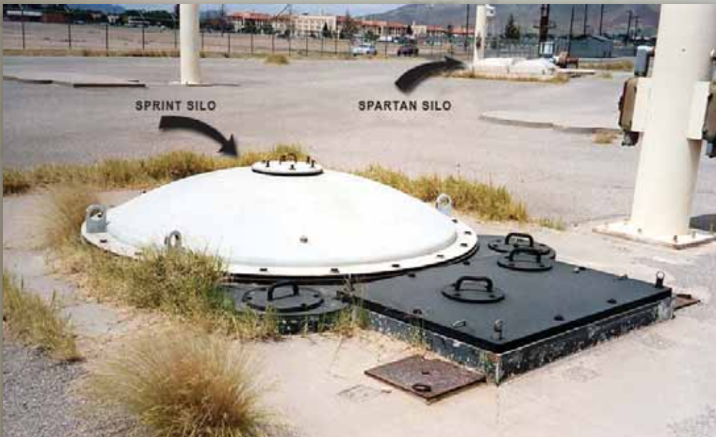
Sprint silo (foreground) and Spartan silo (background) at the Safeguard Central Training Facility. Part of the five silo mock launch station
