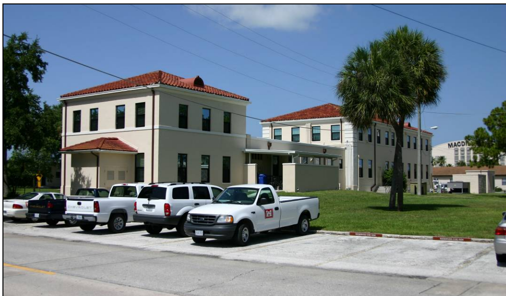
Figure 4-17. Building 26 (Communications Building with Fire Station), MacDill AFB.
