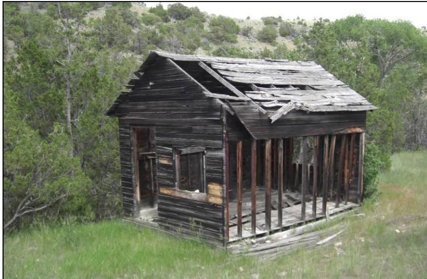
Figure 4-8. CCC cabin constructed on National Forest land now occupied by Montana ARNG as a training area.
