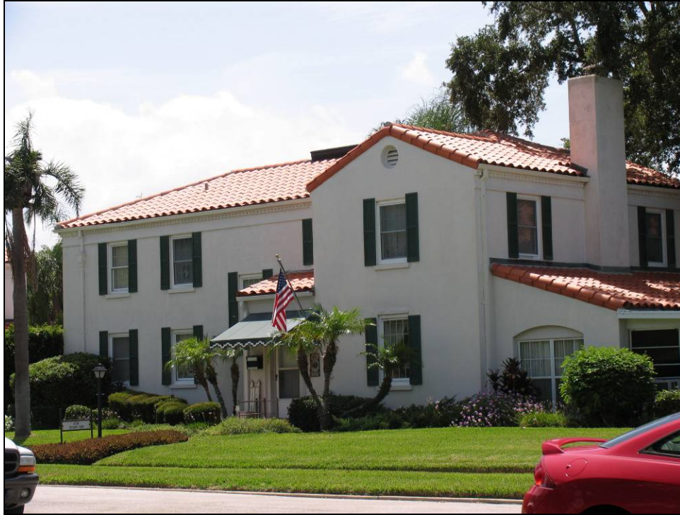
Figure 4-15. Building 404, Staff Circle, MacDill AFB.
