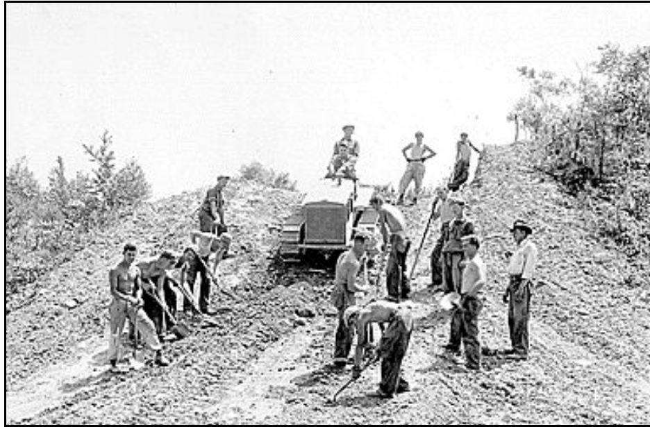
Figure 2-6. CCC Work Crew on Road Construction Project.
