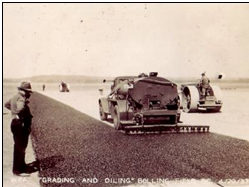
Figure 3-4. Grading and Oiling Runways, Bolling Field, Washington, D.C.
