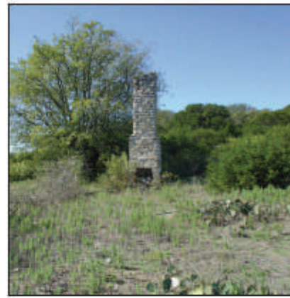
A chimney from a historic structure recalls the past at Fort Hood.
