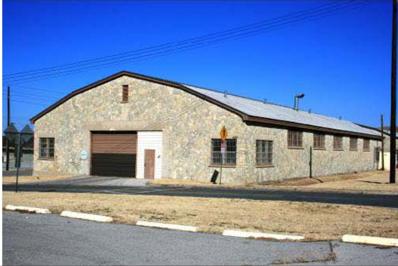
GUN SHED (BLDG 1507) SOUTH AND EAST FACADES, CAMERA FACING NW
