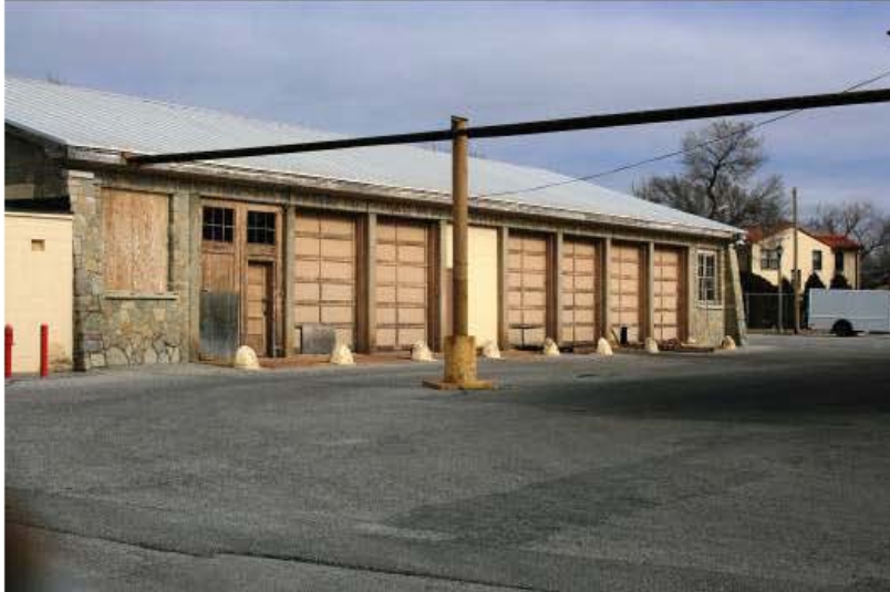
TOP AND BODY SHOP (BLDG 2037), SOUTH FAÇADE, CAMERA FACING NE
