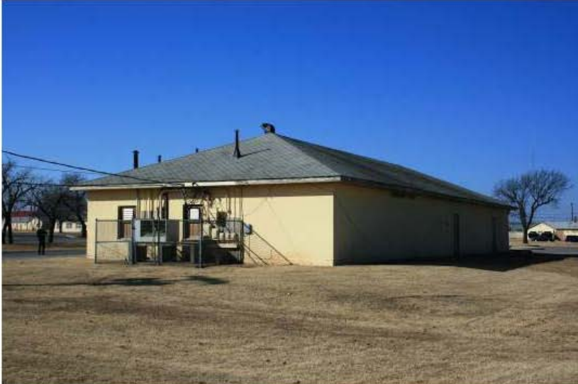
HOSTESS HOUSE (BUILDING 2943), NORTH AND EAST FACADES, CAMERA FACING SW
