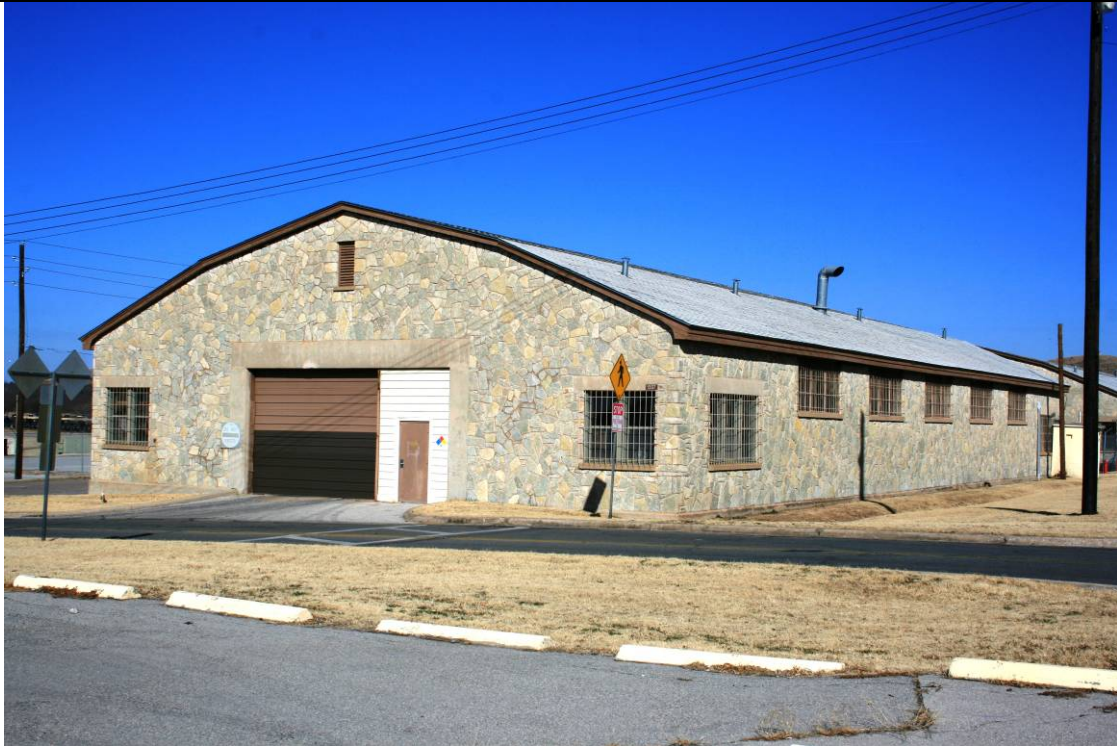
Figure 4-4. Building 1507, Gun Shed
