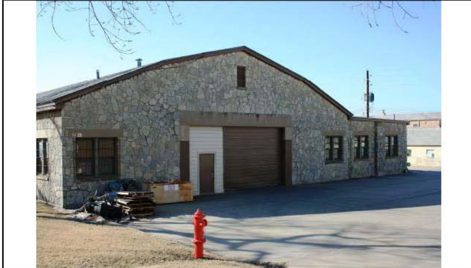
GUN SHED (BLDG 1506), NORTH FAÇADE, CAMERA FACING SW
