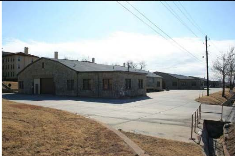
GUN SHED (BLDG 1505) NORTH AND WEST FACADES, CAMERA FACING SE
