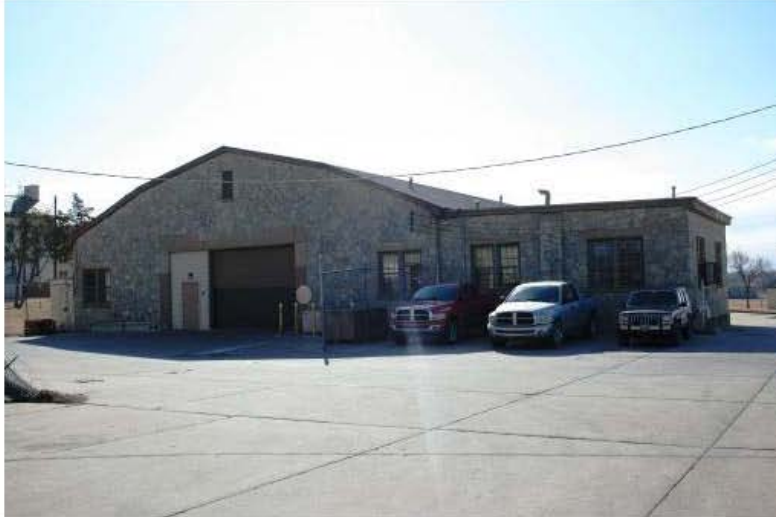
GUN SHED (BLDG 1507) NORTH FAÇADE, CAMERA FACING SSE
