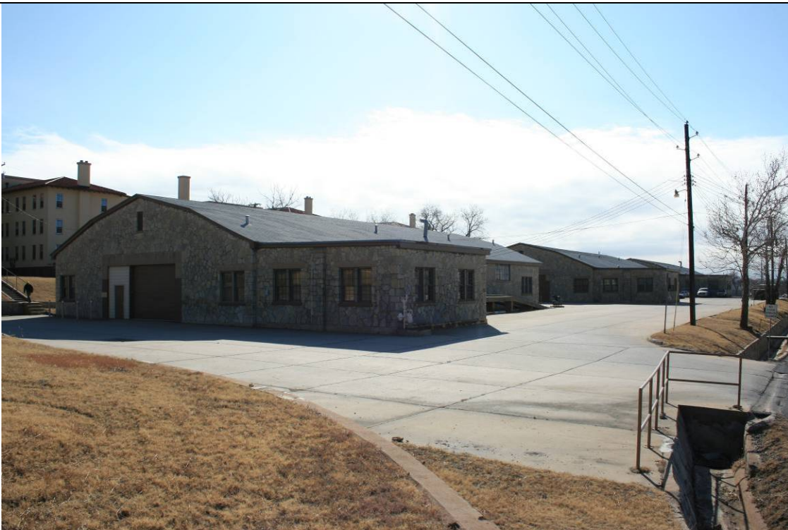
Figure 4-5. Rear of Buildings 1505, 1506, and 1507
