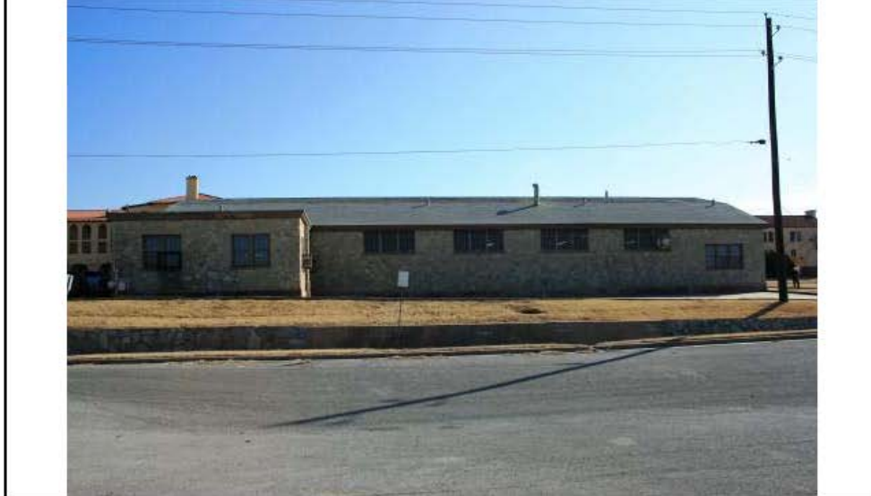
GUN SHED (BLDG 1506), WEST FAÇADE, CAMER FACING EAST
