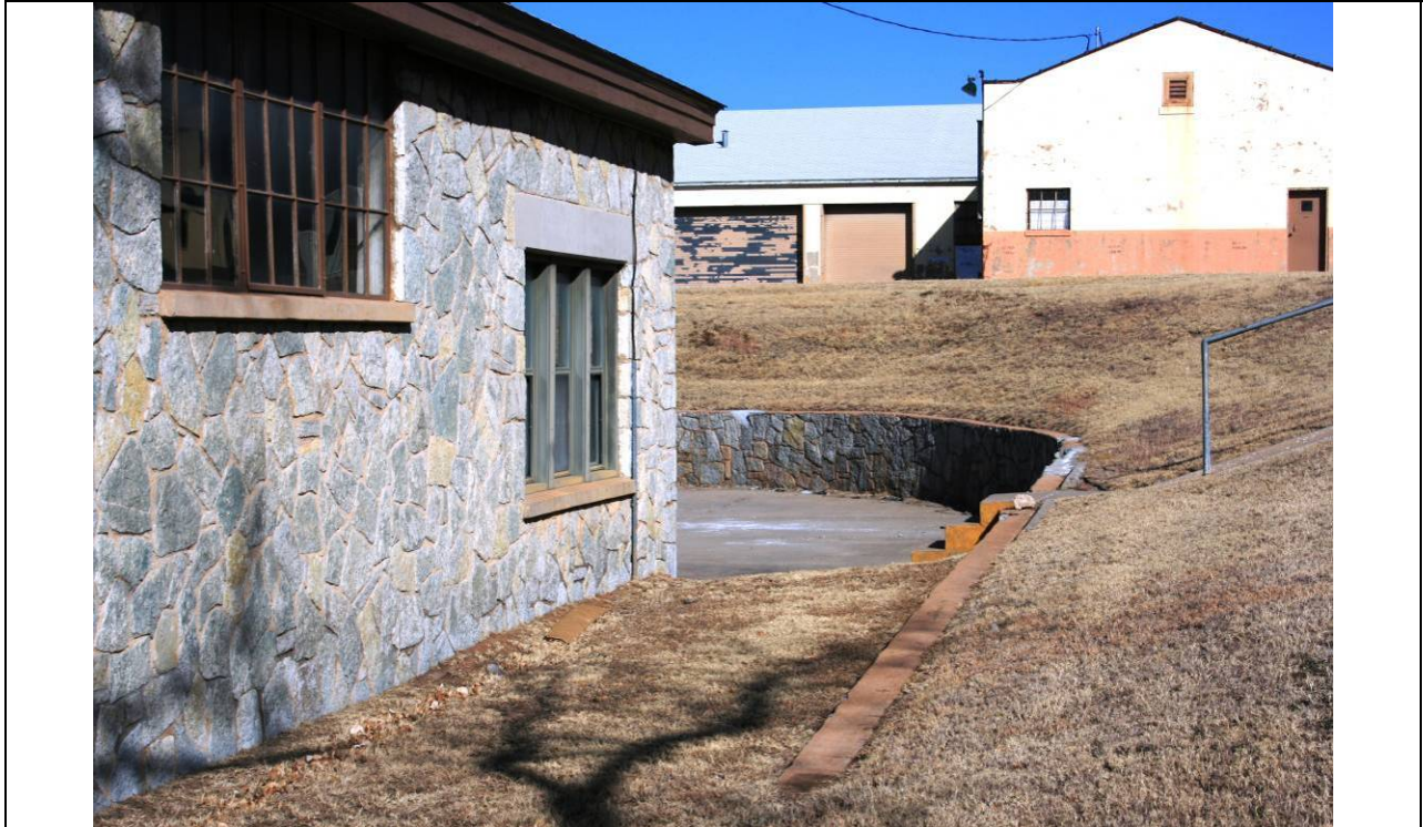
Figure 4-6. Retaining wall at rear of Building 1505
