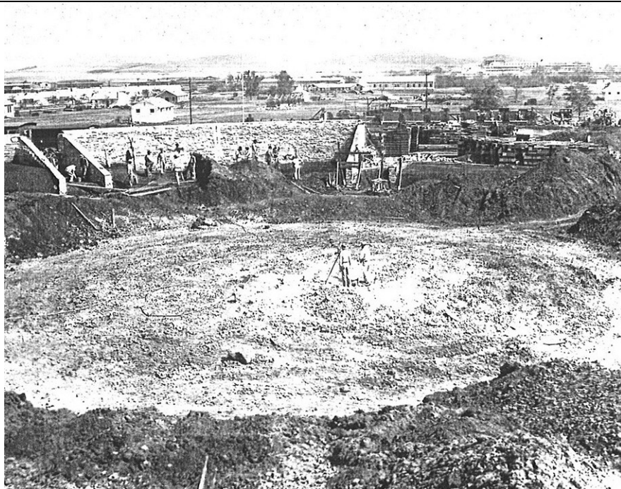
Figure 3-2. Artillery Bowl under construction (Fort Sill National Historic Landmark & Museum).
