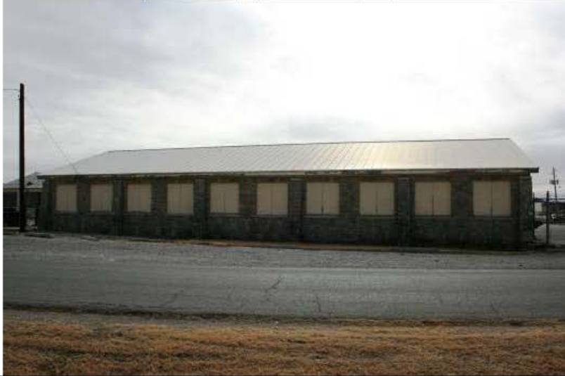
TOP AND BODY SHOP (BLDG 2037), NORTH FAÇADE, CAMERA FACING S
