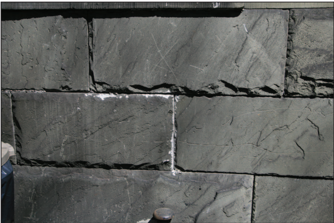
Example of Spalling Granite Arrises
