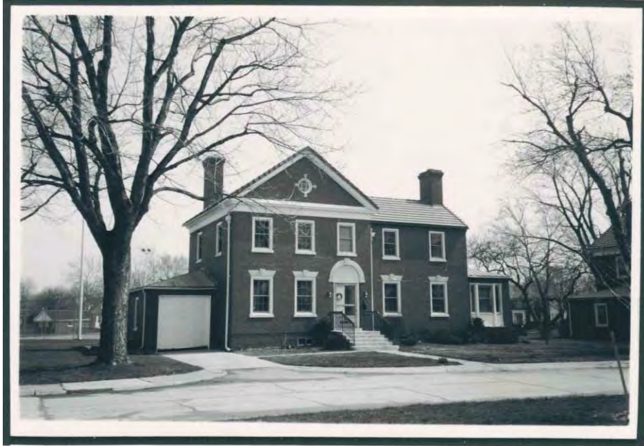
Figure 4. 1935 Georgian Colonial Revival officer quarters at Selfridge Air National Guard Base, Michigan. (Photo taken by RCG&A)
