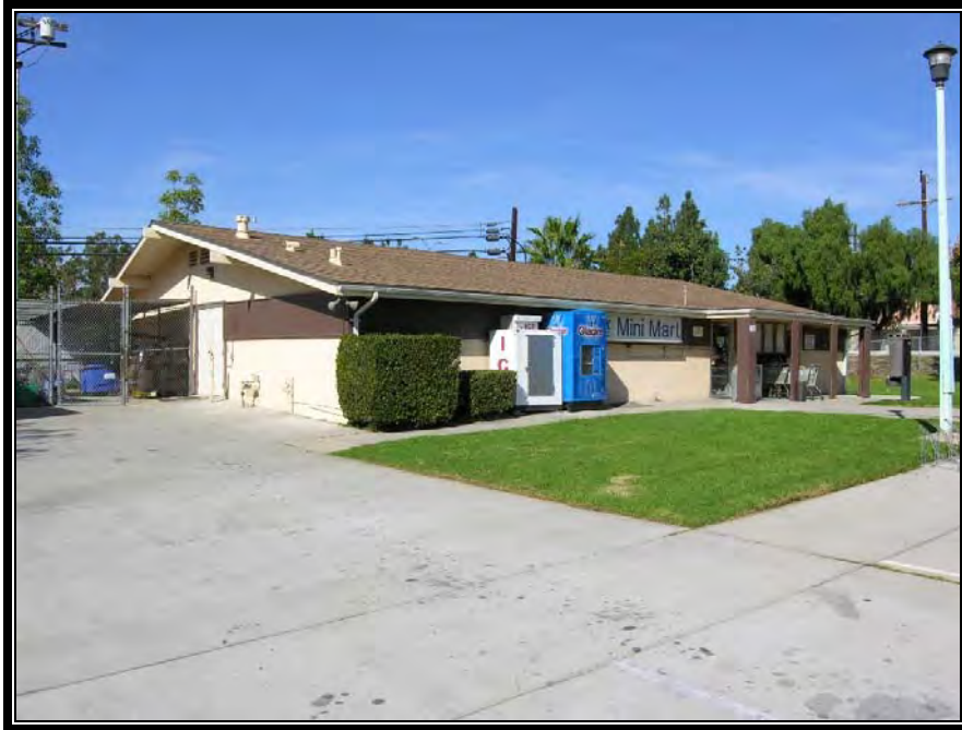
Figure A.1.50. “Mini Mart,” Catalina Heights (Capehart housing), NBVC, California, 2005. (Photo taken by RCG&A)
