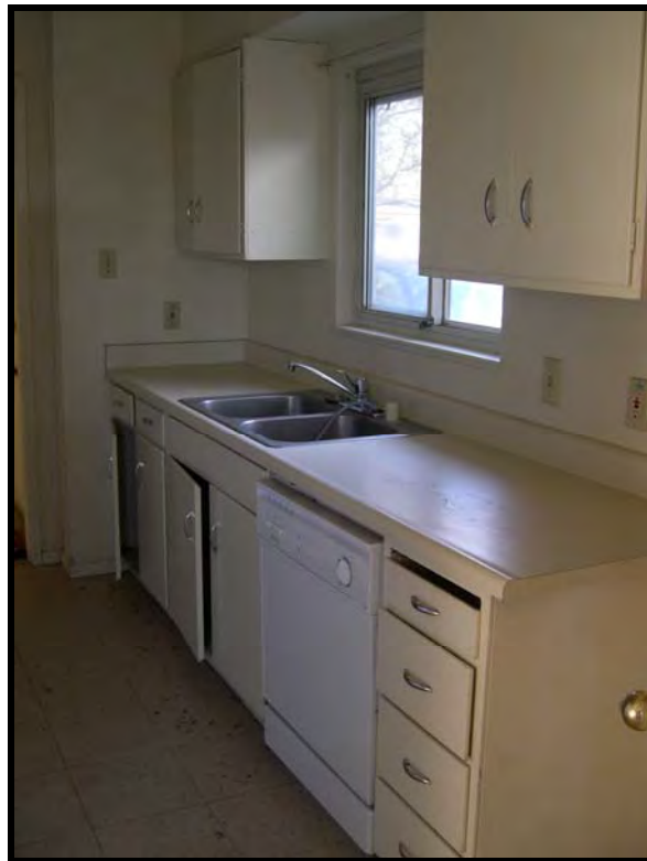
Figure A.5.27. 103 Armstrong Street kitchen (Type 4A1, New Capehart housing), Travis AFB, California, 2005. (Photo taken by RCG&A)
