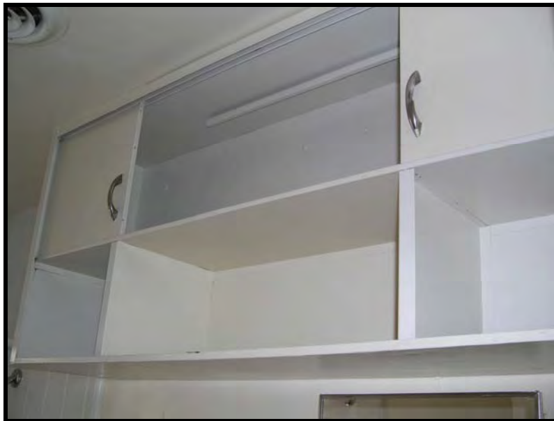
Figure A.2.8. 8010 Corsair Drive bathroom medicine cabinet (Wherry housing), NSA Mid-South, Tennessee, 2005. (Photo taken by RCG&A)
