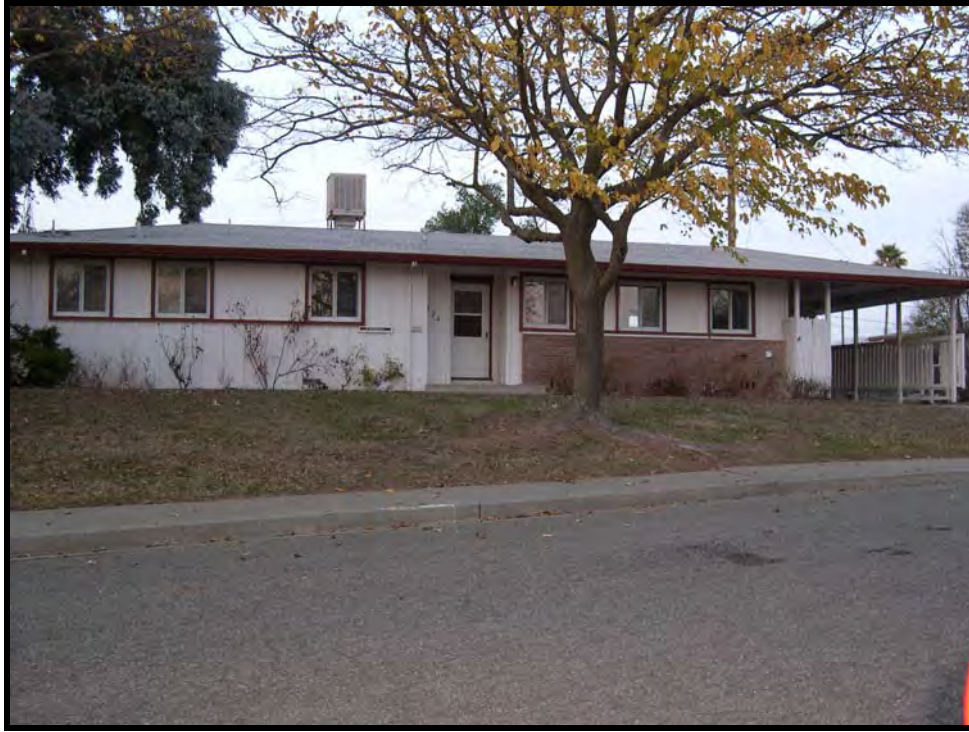
Figure A.5.20. 124 Cannon Drive (Type O-4, 48 Capehart housing), Travis AFB, California, 2005. (Photo taken by RCG&A)
