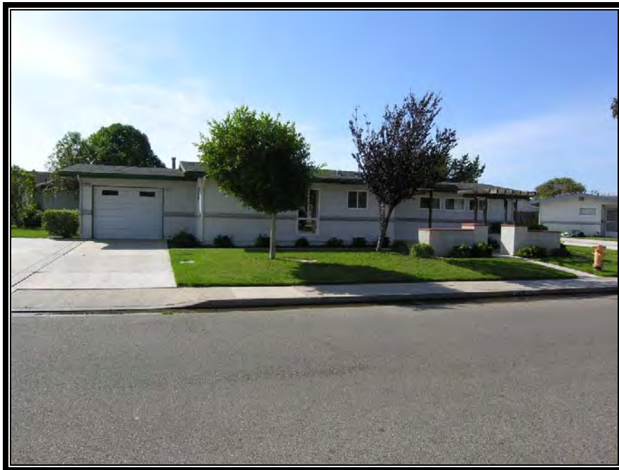
Figure A.1.19. Plan 1A single-family unit (1419 Regulus Drive), Santa Rosa (Capehart housing), NBVC, California, 2005. (Photo taken by RCG&A)
