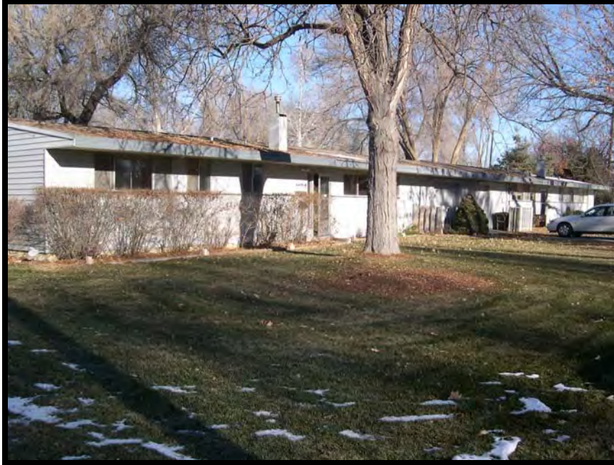
Figure A.4.14. 4475B Tuck Street, Mountain Home AFB, Idaho, 2005. (Photo taken by RCG&A)
