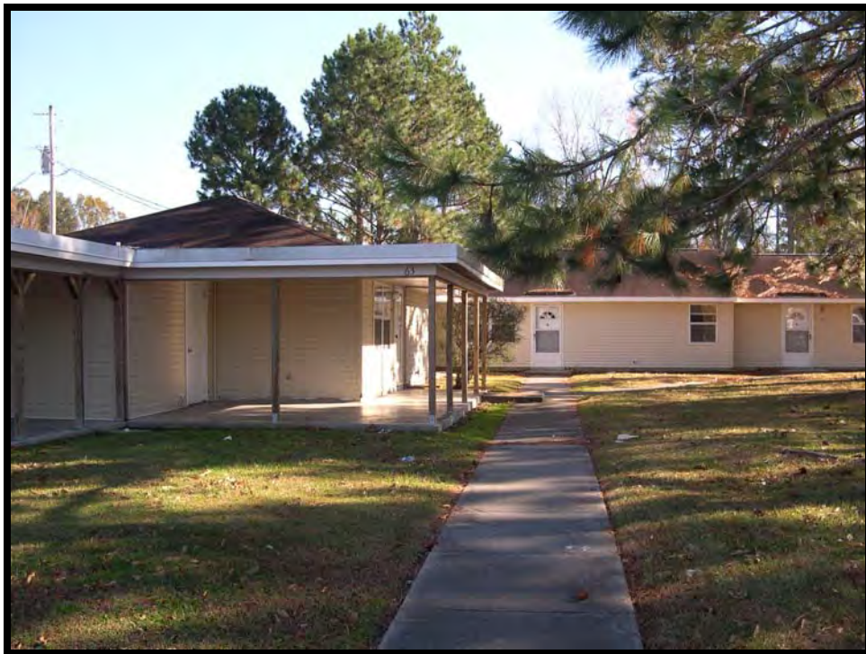
Figure A.3.5. 65-63 Fort Macon Street, Fort Macon (Wherry housing), MCAS Cherry Point, North Carolina, 2005. (Photo taken by RCG&A)
