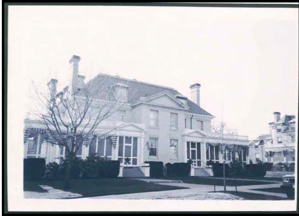
Figure 11. 1905 duplex officers housing designed by Ernest Flagg, U.S. Naval Academy, Maryland. (Photo taken by RCG&A)
