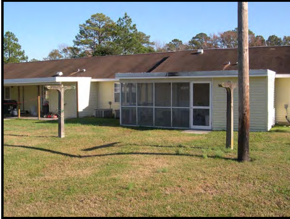
Figure A.3.11. Fort Macon (Wherry housing) rear yards, MCAS Cherry Point, North Carolina, 2005. (Photo taken by RCG&A)
