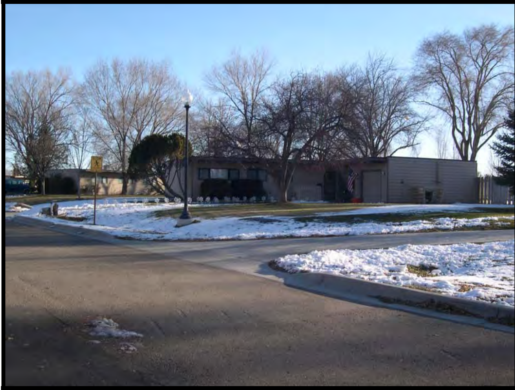
Figure A.4.33. 42 Walnut Street, Mountain Home AFB, Idaho, 2005. (Photo taken by RCG&A)
