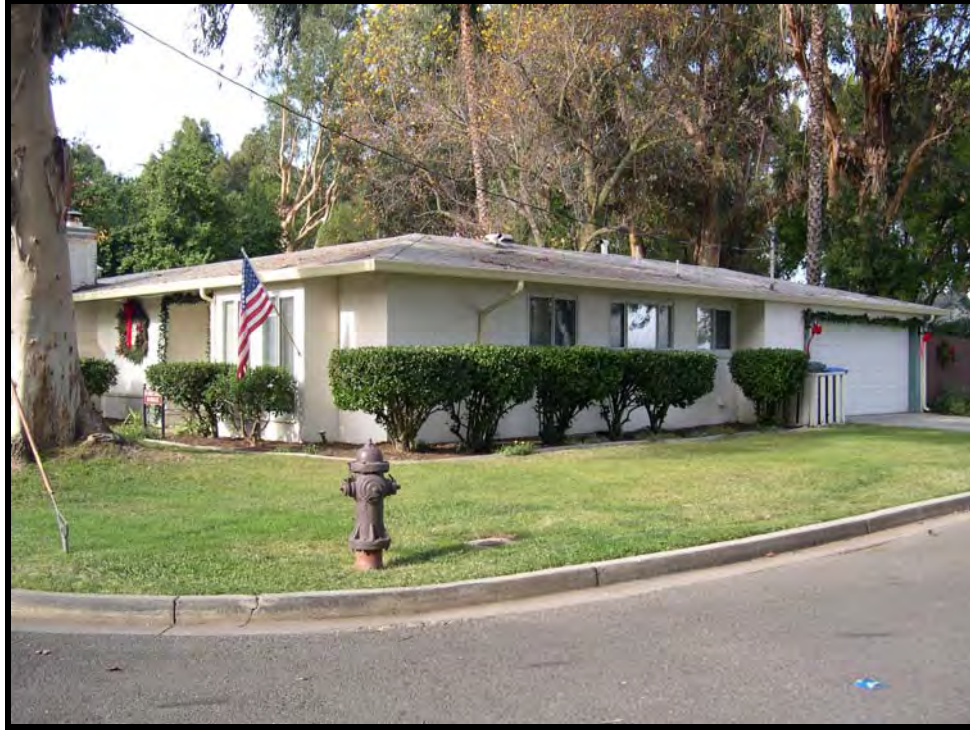
Figure A.5.41. 904 Luke Street side elevation (General, Appropriated Funds housing), Travis AFB, California, 2005. (Photo taken by RCG&A)
