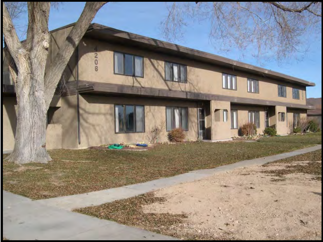
Figure A.4.7. Building 4206, Mountain Home AFB, Idaho, 2005. (Photo taken by RCG&A)
