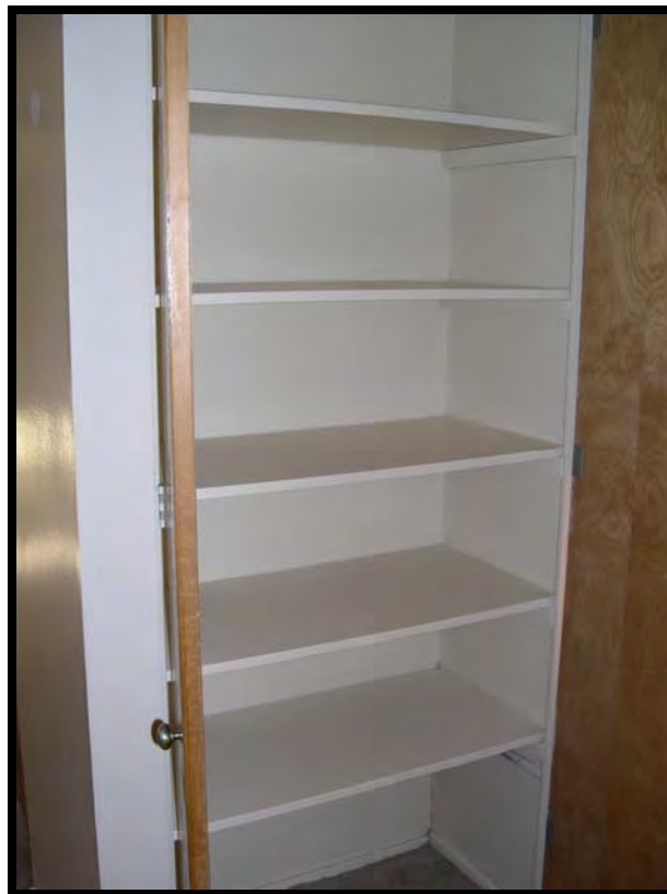
Figure A.4.15. 4475B Tuck Street hall linen closet, Mountain Home AFB, Idaho, 2005. (Photo taken by RCG&A)
