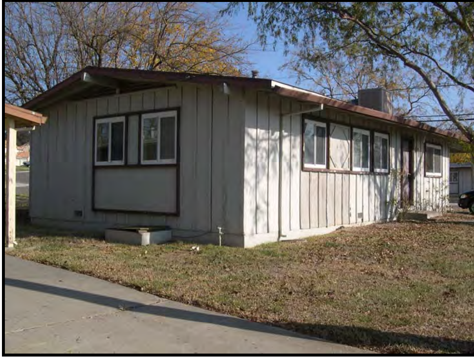
Figure A.5.9. 381 Fairchild Drive front elevation (Type A-1, Old Capehart housing), Travis AFB, California, 2005. (Photo taken by RCG&A)
