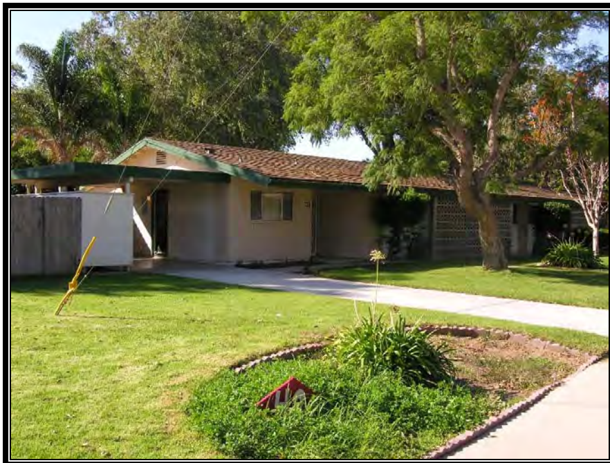
Figure A.1.43. Duplex unit (Building 1012), Catalina Heights (Capehart housing), NBVC, California, 2005. (Photo taken by RCG&A)
