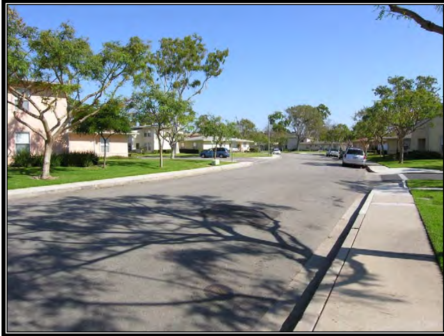
Figure A.1.5. Perry Drive, Bruns Park (Wherry housing), NBVC, California, 2005. (Photo taken by RCG&A)
