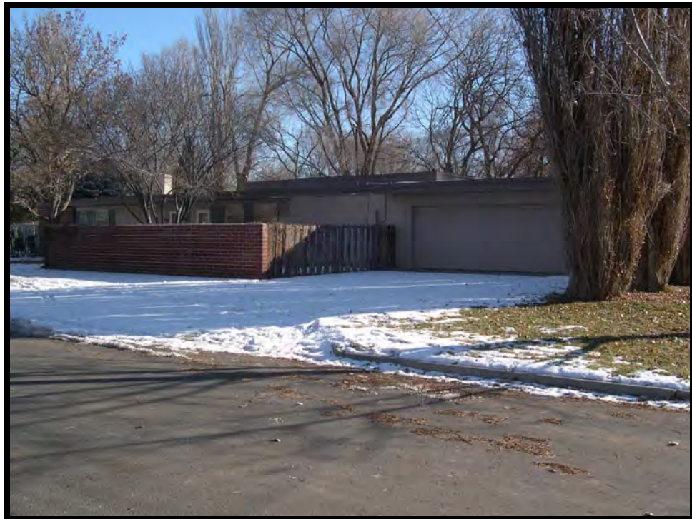
Figure A.4.19. 4478 Tuck Street front elevation (Colonel, Old Capehart housing), Mountain Home AFB, Idaho, 2005. (Photo taken by RCG&A)
