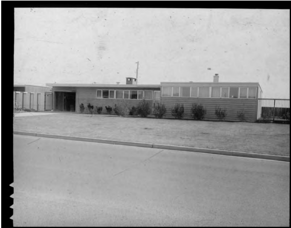
Figure 25: Senior Officer quarters (Wherry housing), Mountain Home AFB, Idaho, ca. 1956. (Courtesy of Cultural Resources Manager, Mountain Home AFB)
