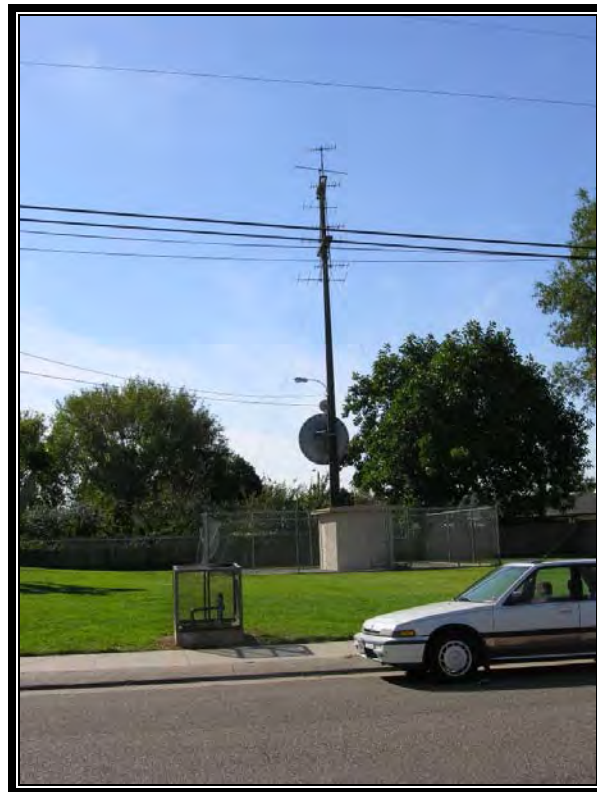
Figure A.1.51. Master TV antenna, Catalina Heights (Capehart housing), NBVC, California, 2005. (Photo taken by RCG&A)
