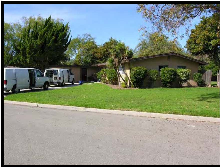
Figure A.1.26. Plan 14AR single-family unit (1001 Polaris Drive), Santa Rosa (Capehart housing), NBVC, California, 2005. (Photo taken by RCG&A)
