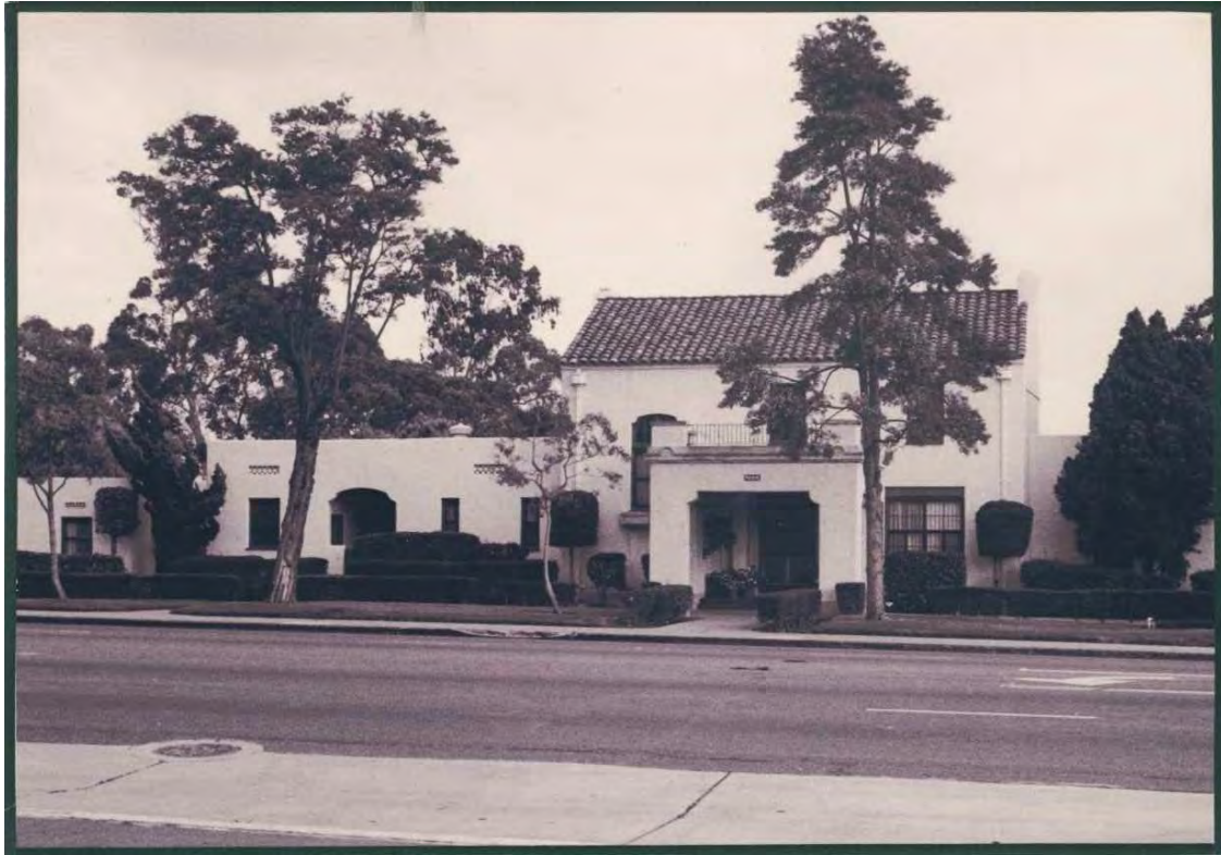
Figure 12. 1922 senior officer housing (Quarters A) at Naval Training Center, San Diego, California. (Photo taken by RCG&A)
