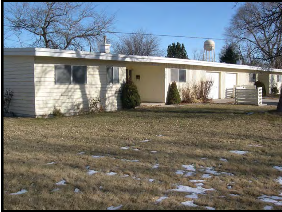
Figure A.4.23. 4759A Tamarack Street front elevation (Type 1-A-2, New Capehart housing), Mountain Home AFB, Idaho, 2005. (Photo taken by RCG&A)
