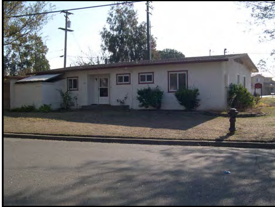
Figure A.5.32. 183 Collins Street front elevation (Type 3M1, New Capehart housing), Travis AFB, California, 2005. (Photo taken by RCG&A)
