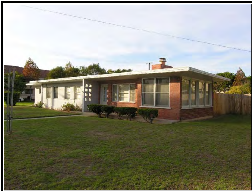
Figure A.1.55. Single-family unit (Building 1132), Port Hueneme (appropriated-funds housing), NBVC, California, 2005. (Photo taken by RCG&A)
