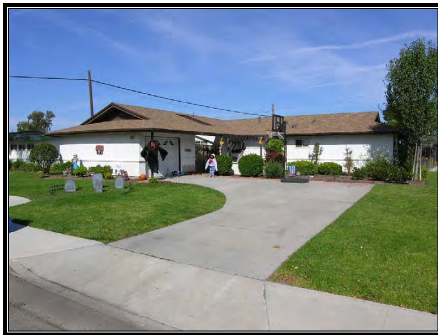
Figure A.1.15. Plan 6C single-family unit (1152 Regulus Drive), Santa Rosa (Capehart housing), NBVC, California, 2005. (Photo taken by RCG&A)
