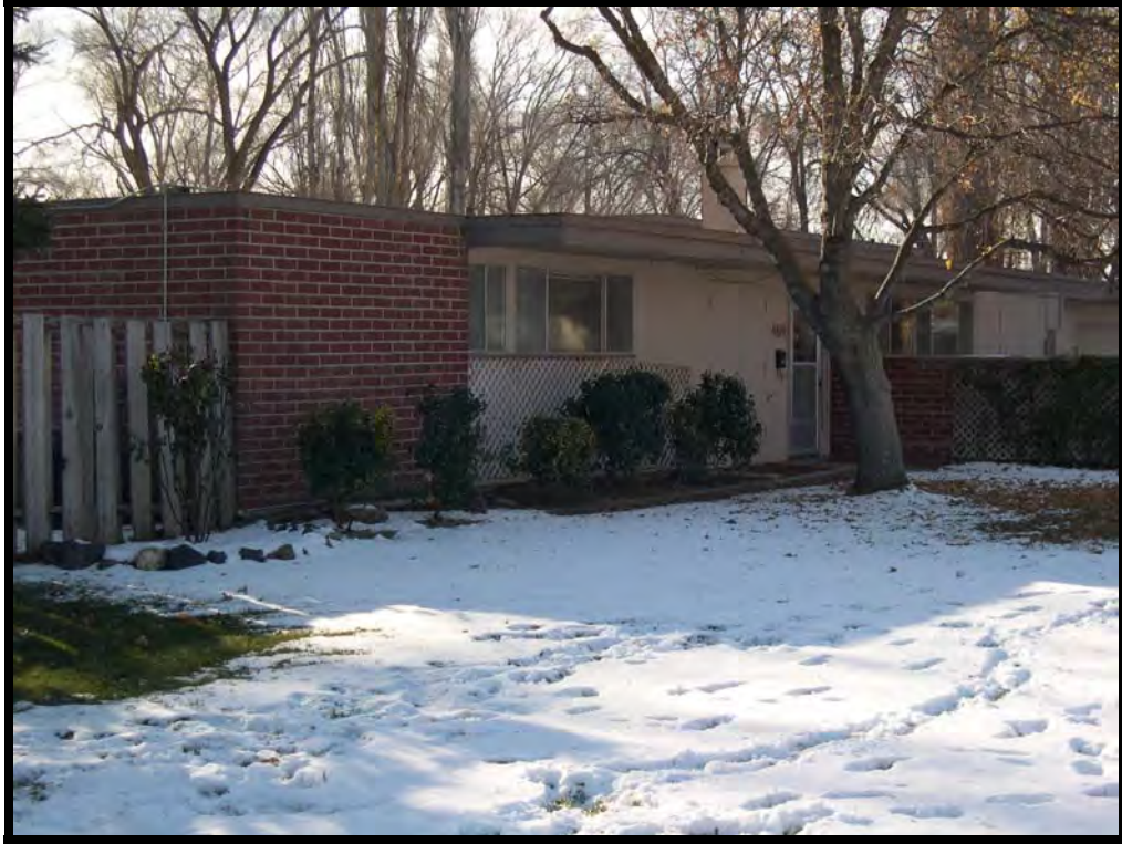
Figure A.4.18. 4478 Tuck Street front elevation, (Colonel, Old Capehart housing), Mountain Home AFB, Idaho, 2005. (Courtesy of Mountain Home AFB, 366 th Civil Engineer Squadron)
