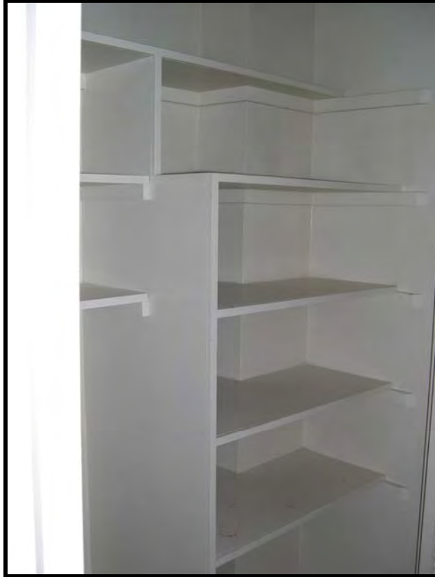
Figure A.2.7. 8010 Corsair Drive built-in closet (Wherry housing), NSA Mid-South, Tennessee, 2005. (Photo taken by RCG&A)
