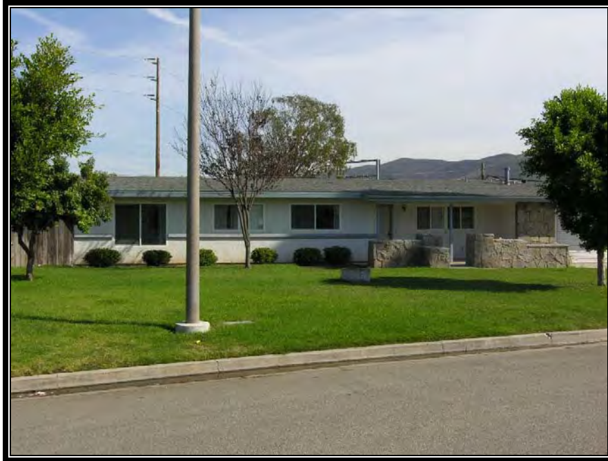
Figure A.1.22. Plan 8A single-family unit (1416 Regulus Drive), Santa Rosa, (Capehart housing) NBVC, California, 2005. (Photo taken by RCG&A)
