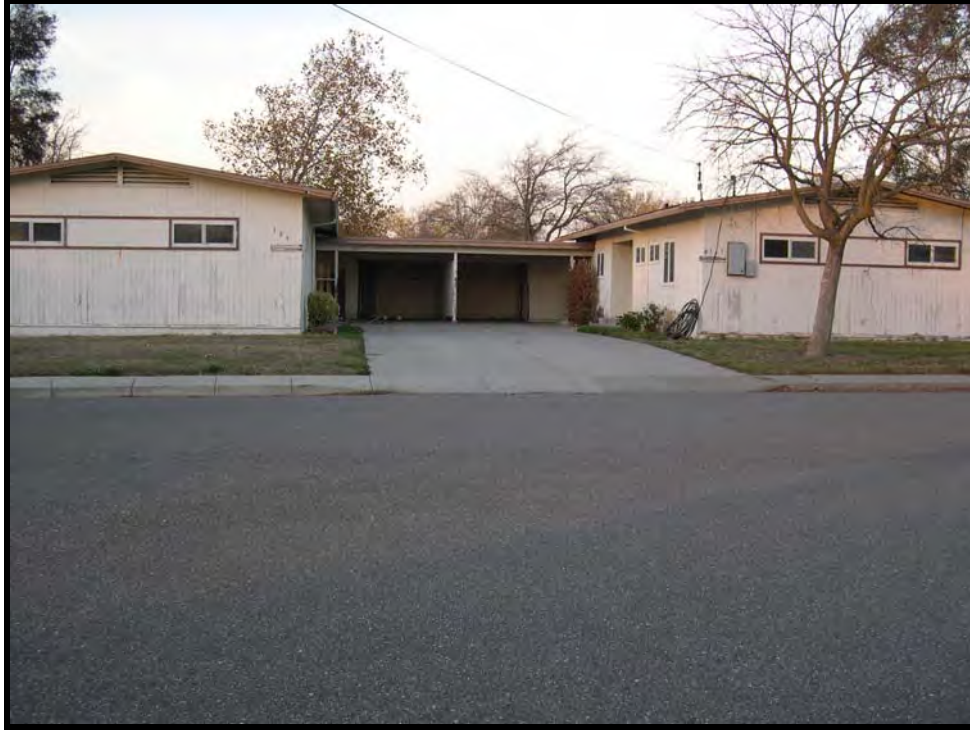
Figure A.5.23. 109-111 Pope Court front elevation (Type 3A1, New Capehart housing), Travis AFB, California, 2005. (Photo taken by RCG&A)
