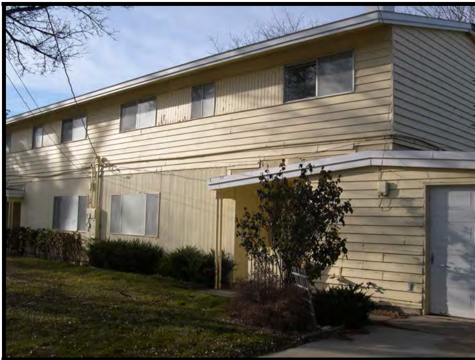
Figure A.4.24. 4757A Buchanan Street front elevation (Type 2-A-2, New Capehart housing), Mountain Home AFB, Idaho, 2005. (Photo taken by RCG&A)
