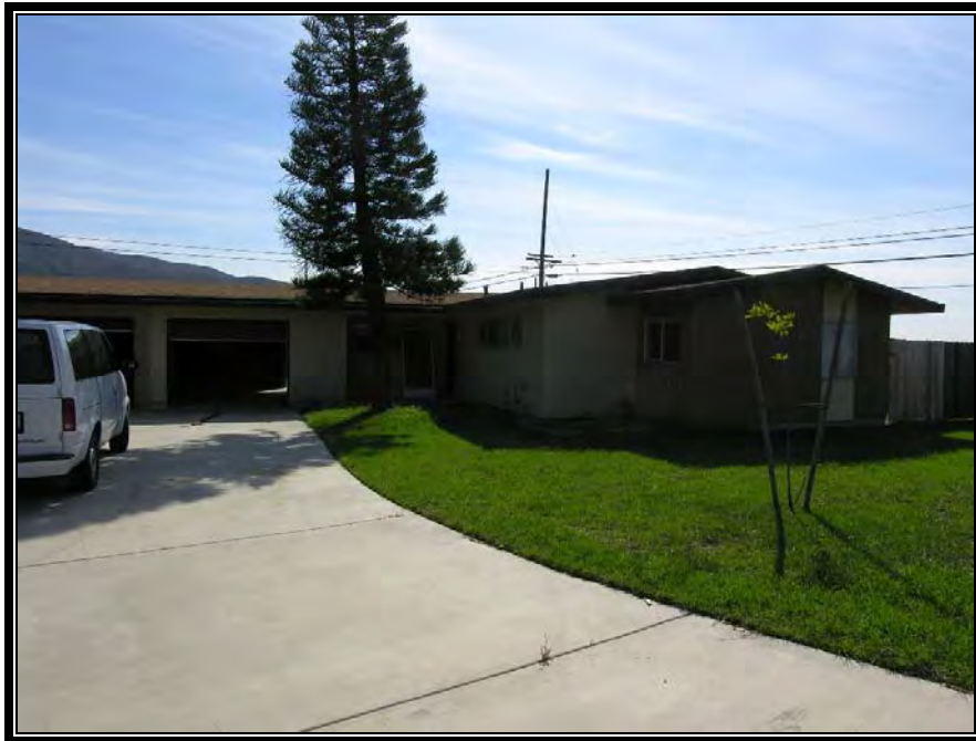
Figure A.1.36. Duplex unit (Building 1987, Unit B), San Miguel (Capehart housing), NBVC, California, 2005. (Photo taken by RCG&A)
