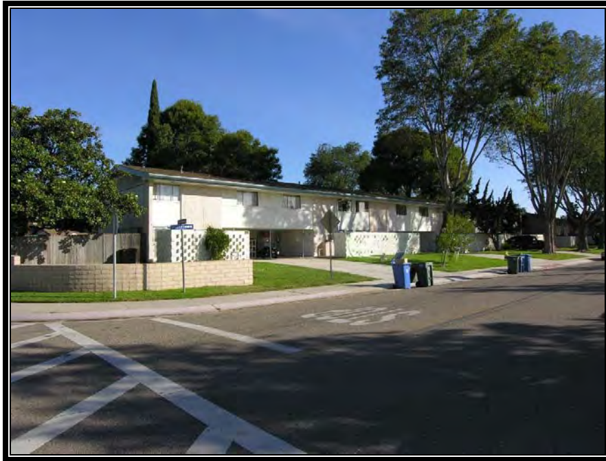
Figure A.1.42. Multi-family unit (Building 1007), Catalina Heights (Capehart housing), NBVC, California, 2005. (Photo taken by RCG&A)
