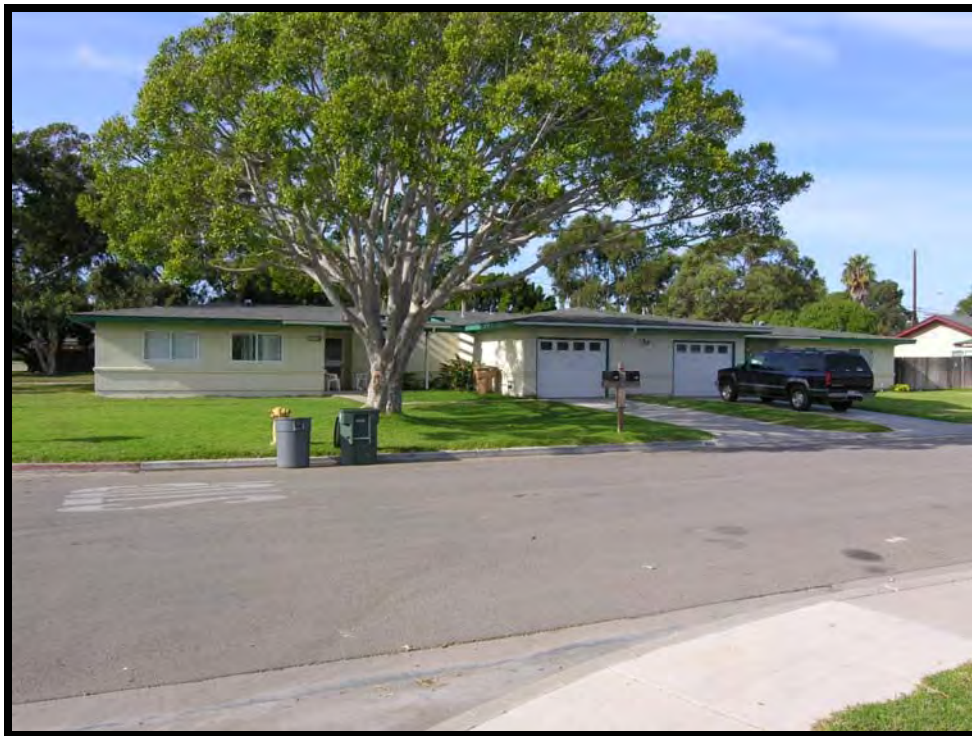
Figure 16: Building 1843, Tartar Drive, San Miguel Neighborhood (Capehart housing), Point Mugu, NBVC, California, 2005. (Photo taken by RCG&A)
