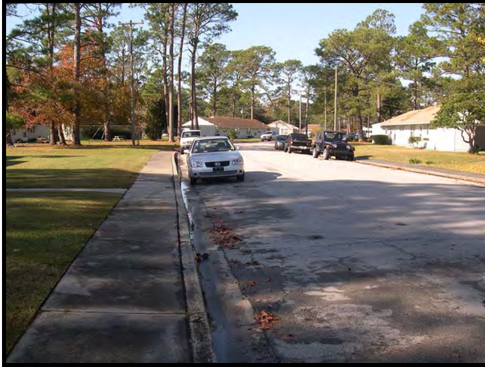
Figure A.3.17. East Moret Drive streetscape, Hancock Village (Wherry housing), MCAS Cherry Point, North Carolina, 2005. (Photo taken by RCG&A)
