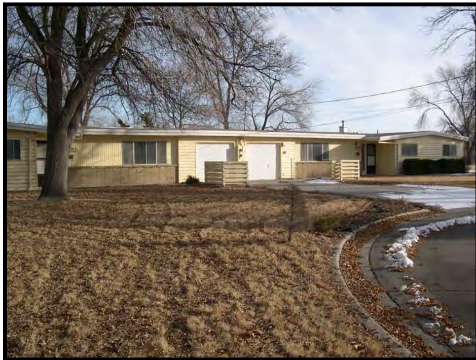
Figure A.4.30. 4647AB Taylor Street front elevation (Type 3-A-2, New Capehart housing), Mountain Home AFB, Idaho, 2005. (Photo taken by RCG&A)
