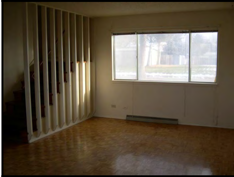
Figure A.4.29. 4757A Buchanan Street living room and stair (Type 2-A-2, New Capehart housing), Mountain Home AFB, Idaho, 2005. (Courtesy of Mountain Home AFB Housing Office)
