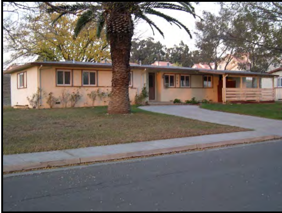
Figure A.5.14. 389 Fairchild Drive front elevation (Type O-10, Old Capehart housing), Travis AFB, California, 2005. (Photo taken by RCG&A)
