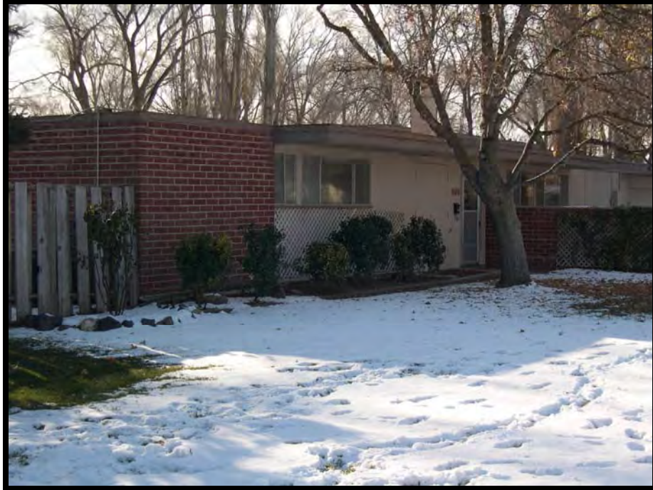
Figure 26: 4478 Tuck Street front elevation, (Colonel, Old Capehart housing), Mountain Home AFB, Idaho, 2005. (Courtesy of Mountain Home AFB, 366 th Civil Engineer Squadron)
