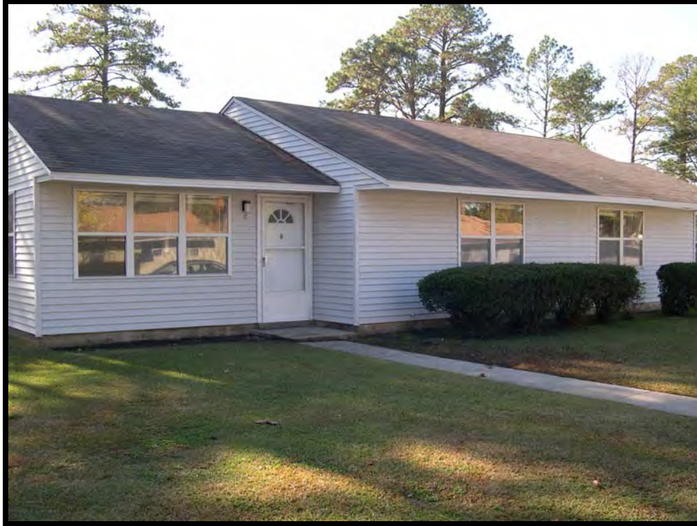
Figure A.3.14. 17 E Moret Drive, Hancock Village (Wherry housing), MCAS Cherry Point, North Carolina, 2005. (Photo taken by RCG&A)
