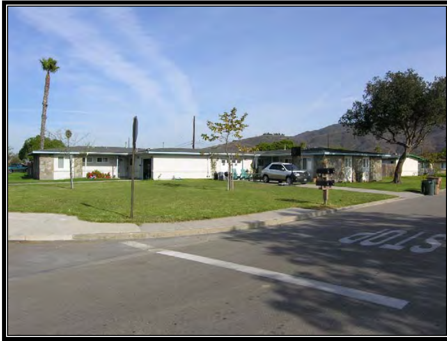
Figure A.1.35. Duplex unit (Building 1902), San Miguel (Capehart housing), NBVC, California, 2005. (Photo taken by RCG&A)
