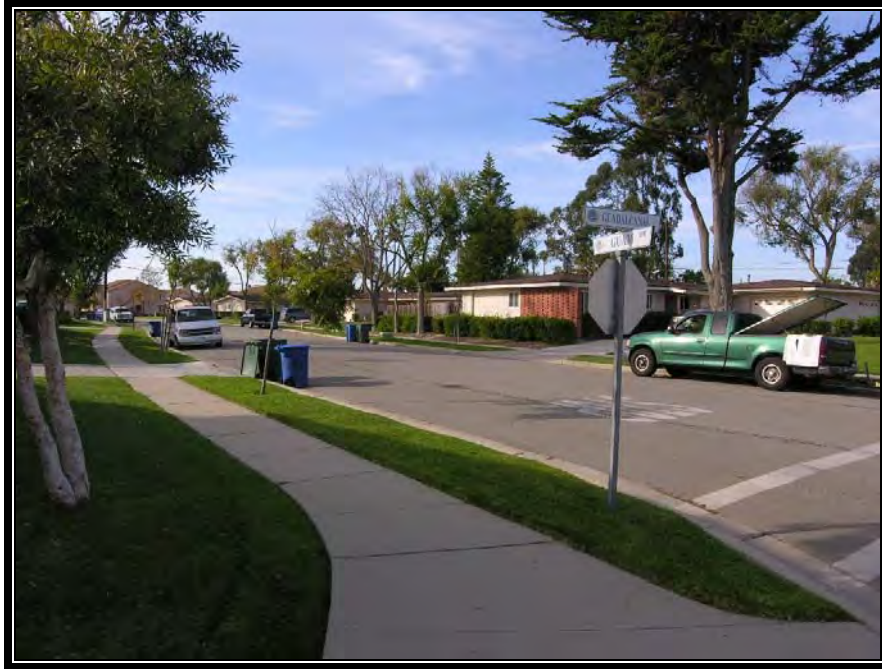
Figure A.1.67. Guam Avenue, Bard Estates (appropriated-funds housing), NBVC, California, 2005. (Photo taken by RCG&A)
