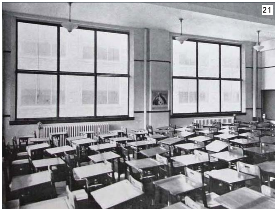
The strength of steel allowed for large expanses of glass that allowed maximum light. This was seen as beneficial in institutional buildings like schools, laboratories, and research facilities.
