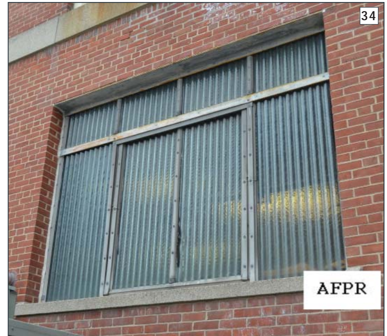
The corrugated wire glass window of Portsmouth Naval Shipyard Building 153 shows the qualities of diffused light and privacy. (Photographer: Kerry Vautrot, 2014)
