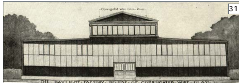
Corrugated wire glass was a dominant building material in the American industrial landscape.
