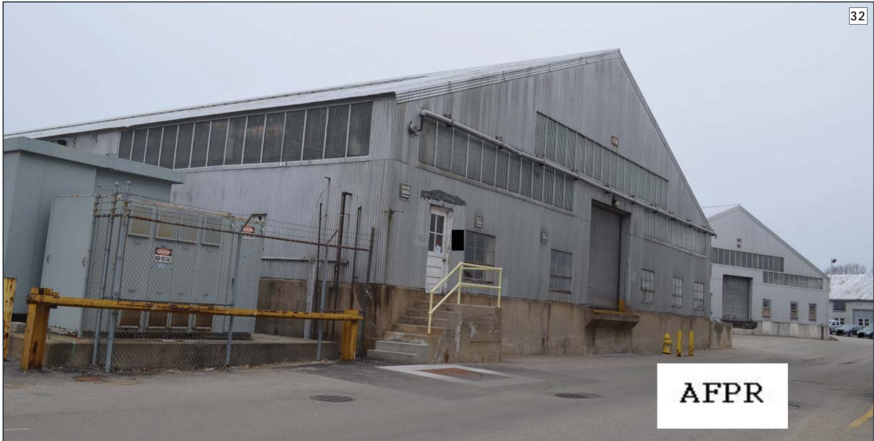
The corrugated wire glass of Portsmouth Naval Shipyard Building 159 is an example of use on a smaller scale. (Photographer: Kerry Vautrot, 2014)
