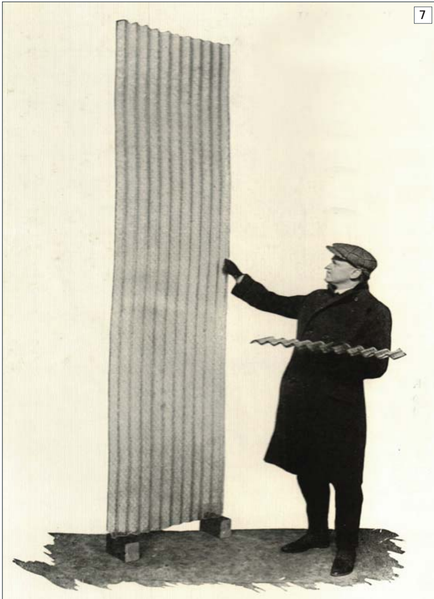
The Hires Turner Glass Company called corrugated wire glass “the lightest and strongest building material of its character obtainable,” and promoted it as the answer to many issues of existing industrial construction. The large panels allowed large expanses of glass without obstruction (left), and the corrugations allowed a much greater load than regular flat glass (right).
