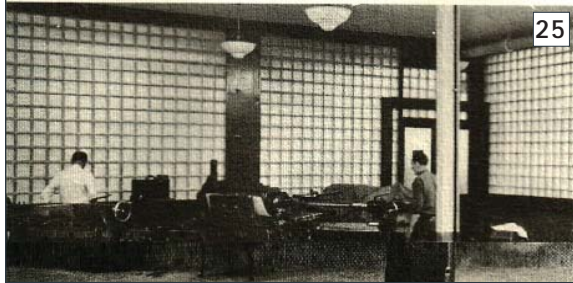
The privacy of glass block walls made it popular for exterior and interior walls of offices, where light was needed but sound was insulated.
