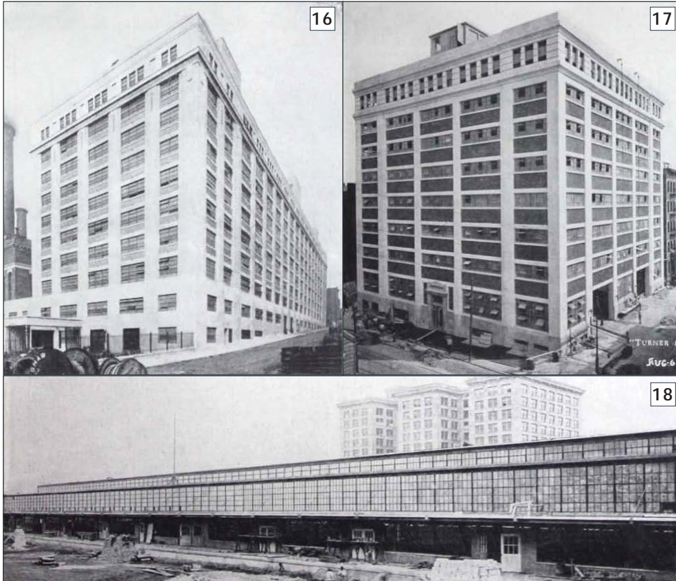
Large steel windows in a series created a distinct change in the architecture of industrial and commercial structures.
