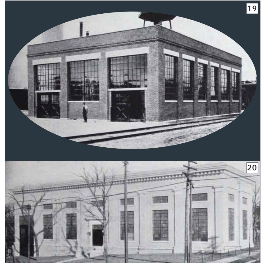
Steel windows could be configured for maximum ventilation, a desirable quality for utilitarian structures like power houses and boiler rooms.
