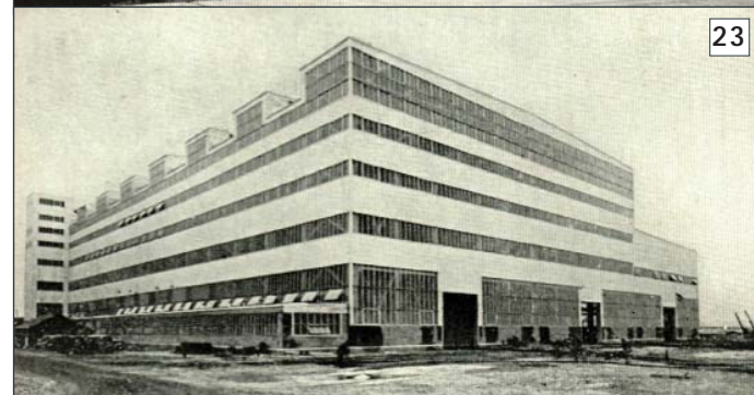
Two examples of the use of corrugated wire glass at the Philadelphia Navy Yard, in the Pipe and Copper Shop (top) and Structural Assembly Shop (bottom).
