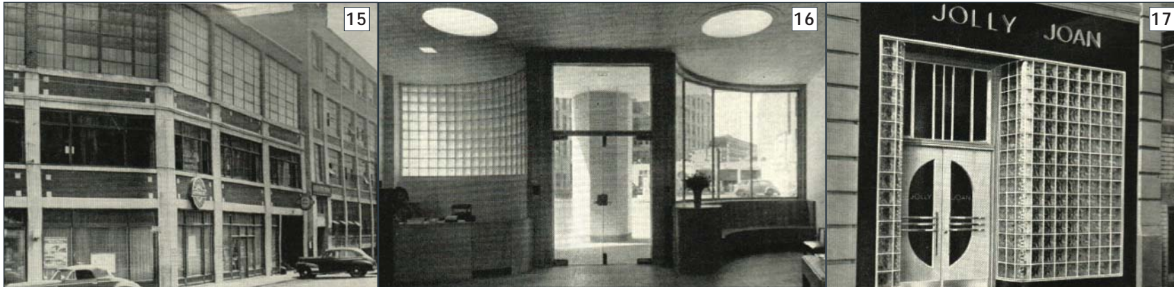
Commercial buildings benefitted from the increased daylight, and glass block was considered the perfect material to show window displays in a natural light.
