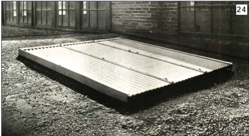
Corrugated wire glass could be used on small-scale projects as well, shown here as a skylight replacement material.
