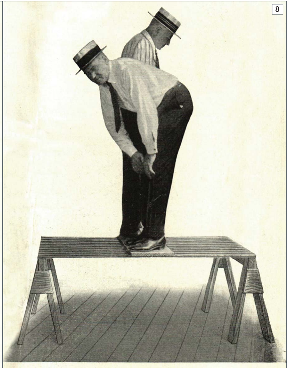
The Hires Turner Glass Company called corrugated wire glass “the lightest and strongest building material of its character obtainable,” and promoted it as the answer to many issues of existing industrial construction. The large panels allowed large expanses of glass without obstruction (left), and the corrugations allowed a much greater load than regular flat glass (right).
