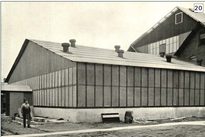
The panels could be a maximum 60" clear span without intermediate support, lending them to be a popular choice for side wall construction.
