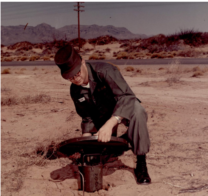
Technician performing maintenance of SOTIM grate and microphone assembly on WSMR. (Date unknown; image courtesy of author)
