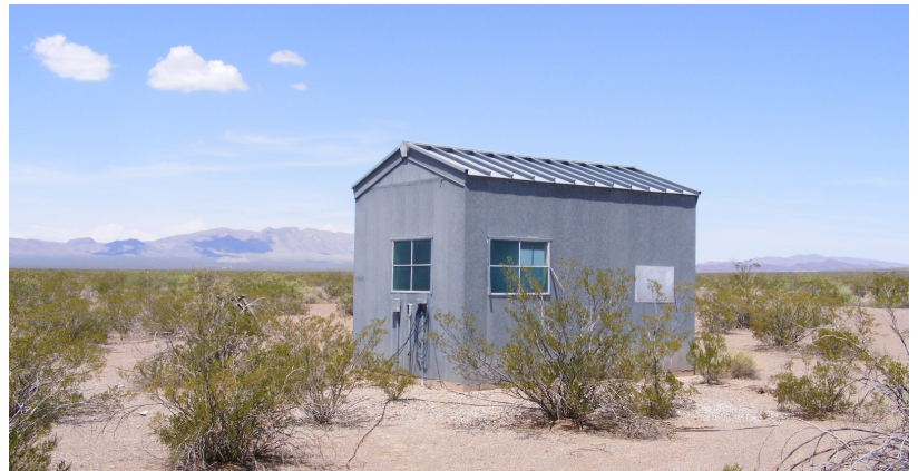
Extant metal building used to house SOTIM data collection equipment on WSMR. (Photo by author)
