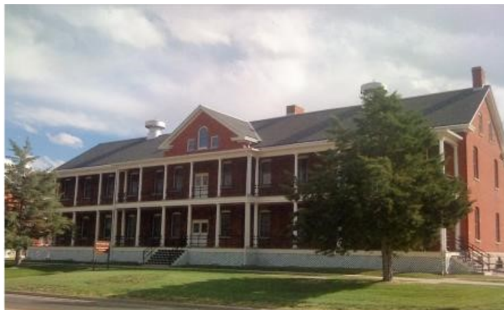
The pre-WWII Enlisted Men's Barracks at F.E. Warren Air Force Base, WY, were constructed between 1905 and 1910. (Image from report)
