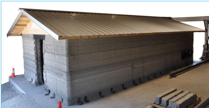
CERL printed concrete building. Source: Ellen Hartman, ERDC-CERL
