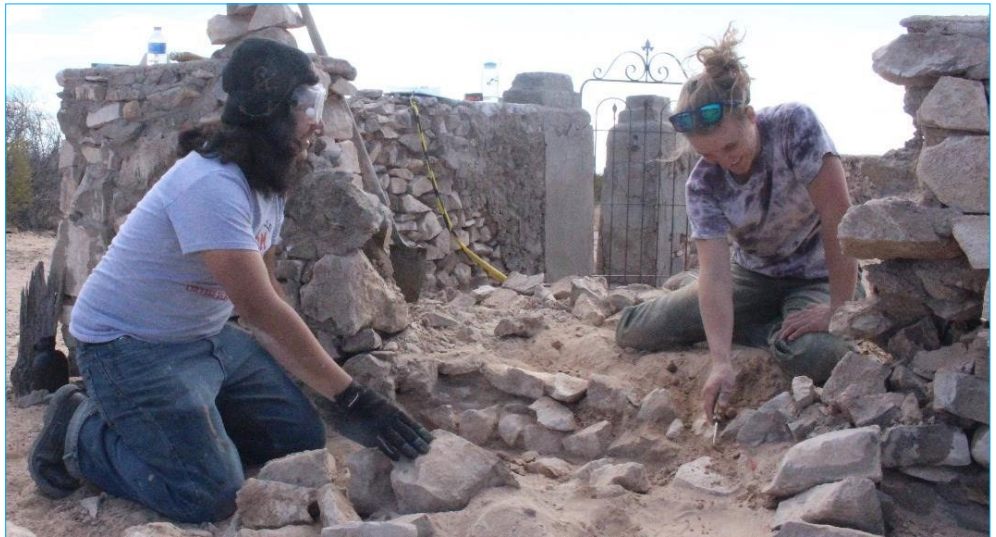
Crew working on repair of perimeter wall. Source: U.S. Army
