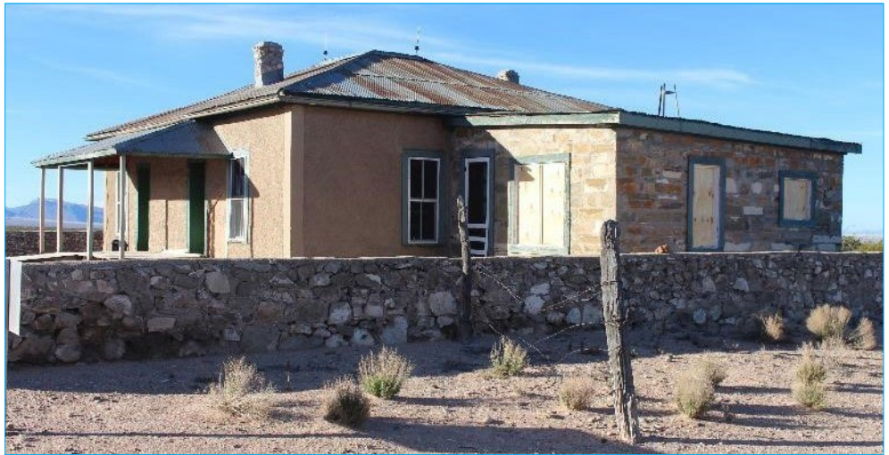
McDonald Ranch house, WSMR. Source: U.S. Army
