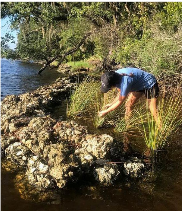
A volunteer helps create a living shoreline to mitigate erosion effects on coastal archaeological sites, Eglin Air Force Base. Source: USAF
