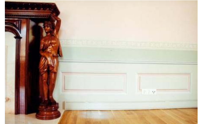
Figure 26 21-1 Baseboard heater panels can be designed to fit within the historic context of the project.
