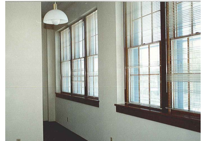
Figure 08 52-2 Installed Back up Windows
