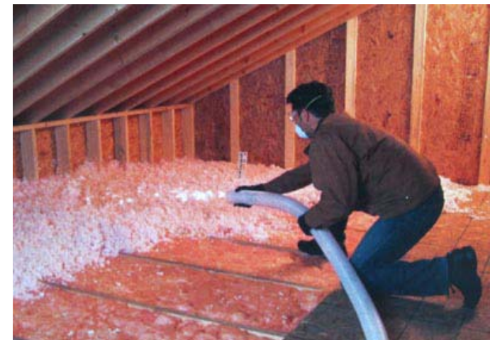
Figure 07 31-5 Blown in Insulation Installation
