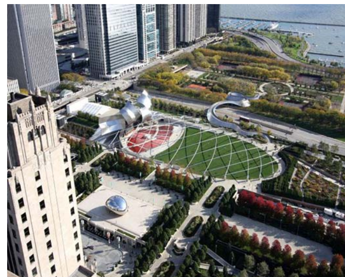
Figure 07 52-5 Intensive Green Roof, Millennium Park, Chicago
