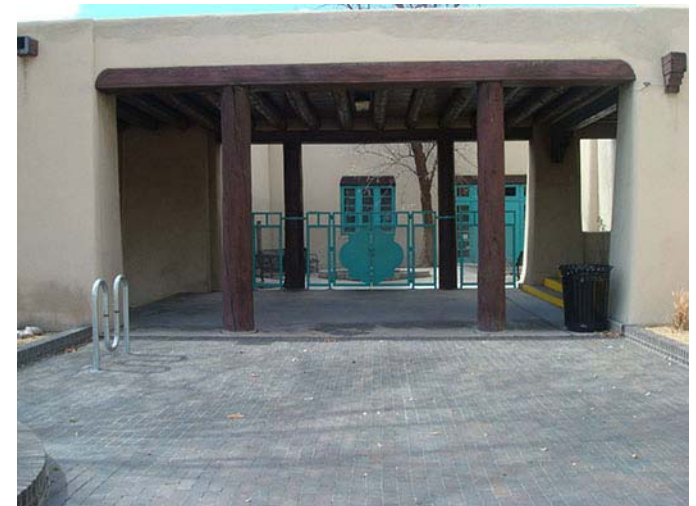
Figure 32 17-5 Dark brick pavers set in sand allow for permeability of water, but absorb and reflect heat from the sun.
