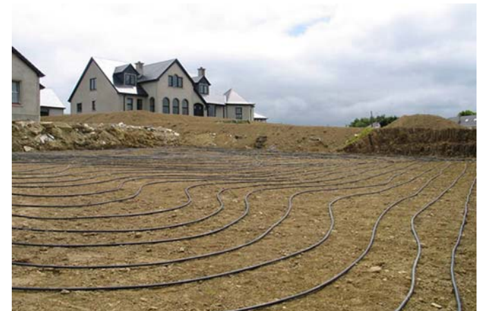
Figure 23 21-2 Closed Loop System
