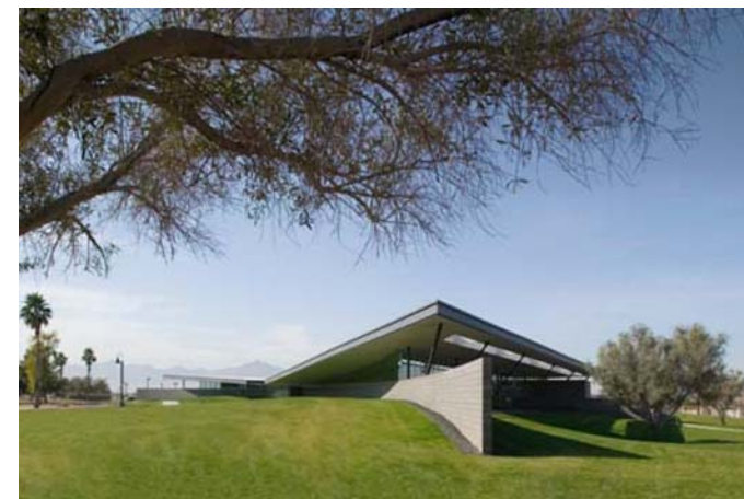
Figure 32 29-7 Earth berms, shown in this photo, provide thermal mass that helps regulate temperatures inside the building. Collected rainwater is used for irrigation.
