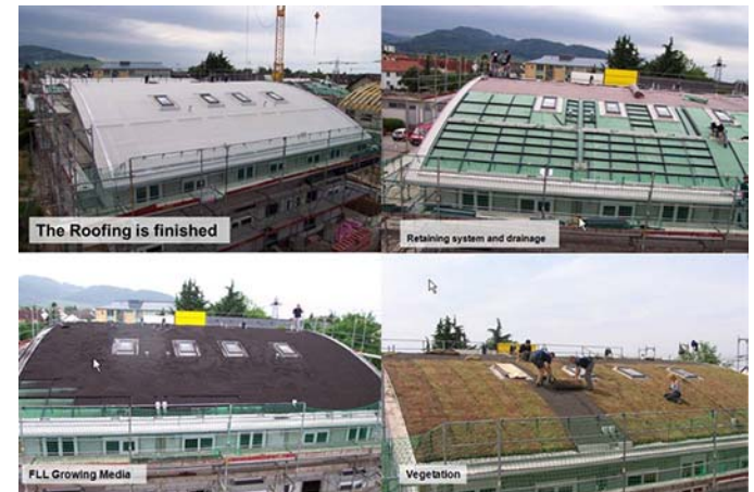
Figure 07 52-8 Installation process on a sloped roof.
