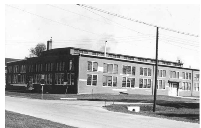
Figure 01 02-7 Atterbury Army Air Field, Columbus, IN. Shop Field Maintenance Building.
