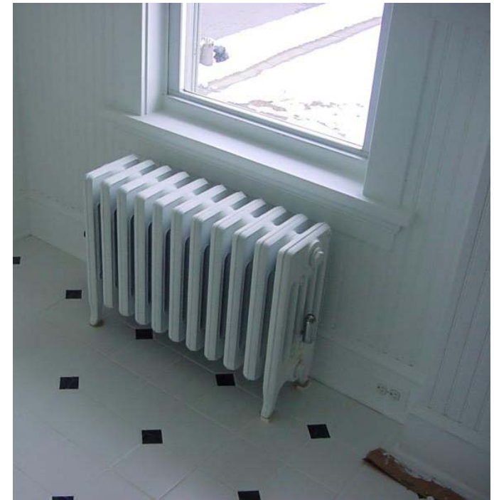
Figure 23 11-3 Radiators are typically located low in the room, like under a window.
