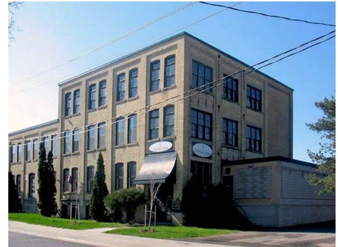
Figure 02 01-28 Office space ventilated with operable windows.
