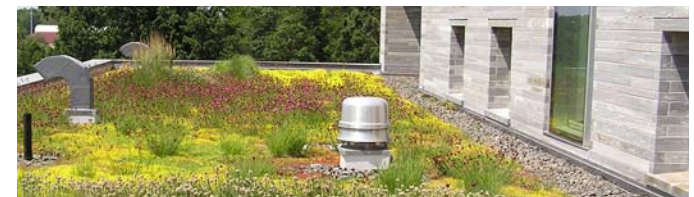
Figure 07 52-3 Extensive green roof
