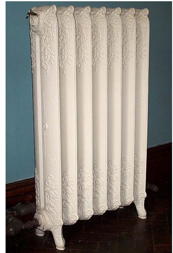
Figure 02 01-18 Decorative Historic Radiator
