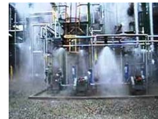
Figure 22 11-11 Deluge Sprinkler System
