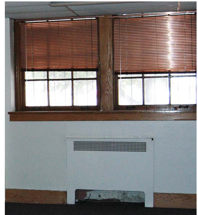
Figure 02 01-16 Decorative radiator cover at Coronado Elementary School, Albuquerque, NM
