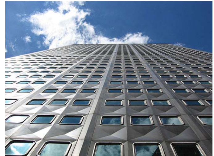
Figure 05 51-11 The Alcoa Building in Pittsburgh, PA (now the Regional Enterprise Tower) was built in 1953. It is a 30 story skyscraper and used 1/8” thick aluminum panels with open, labyrinth-type, pressure-moderating joints.
