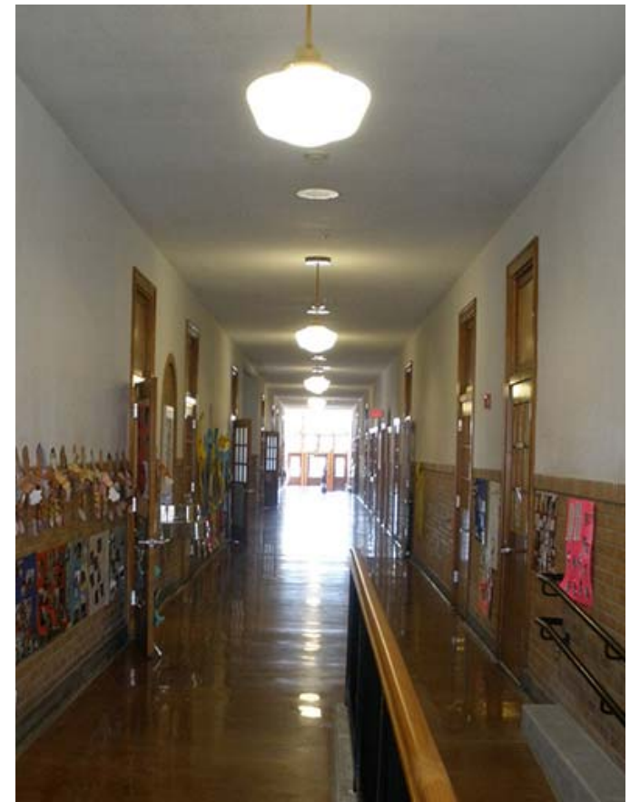
Figure 02 01-31 Transom windows over doors in corridor
