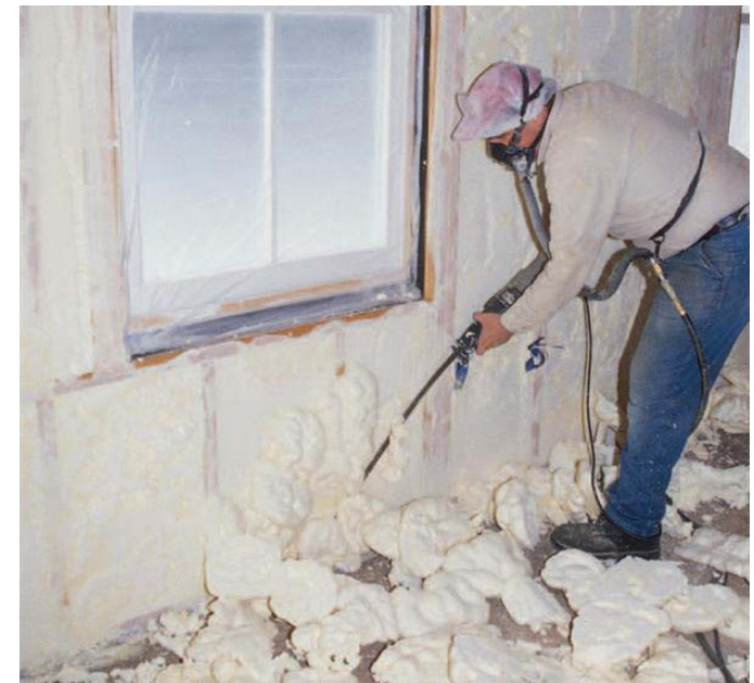
Figure 06 81-11 Trimming is not a feasible option in a Historic Structure
