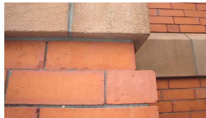
Figure 04 21-2 Repointed Historic brick wall, above
