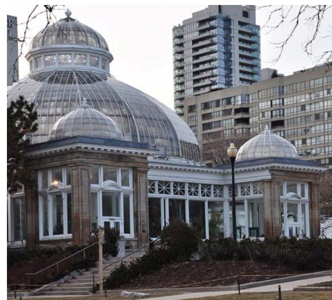
Figure 02 01-22 Commercial Building with glass dome, acting like a sun room.
