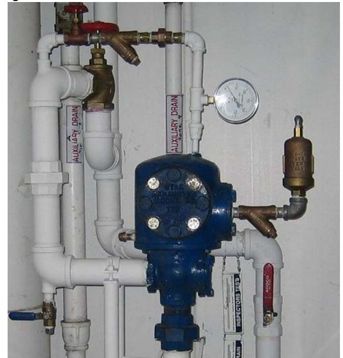
Figure 22 11-7 Dry Pipe System
