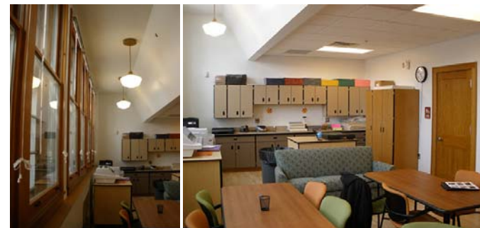
Figure 02 01-24 Figure 02 01-25 After In order to provide well-conditioned space that incorporated the full height of the original windows, gypsum board ceilings formed alcoves near the windows that pulled back to allow for a large portion of acoustical lay-in ceiling tile to be installed in each room.
