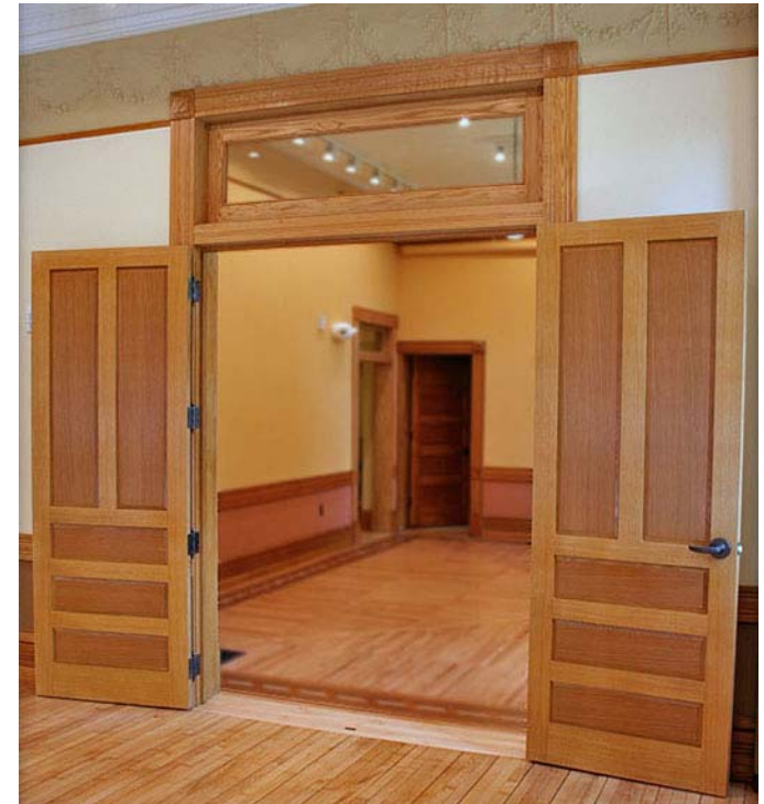
Figure 02 01-3 Transom windows aid in cross-ventilation.
