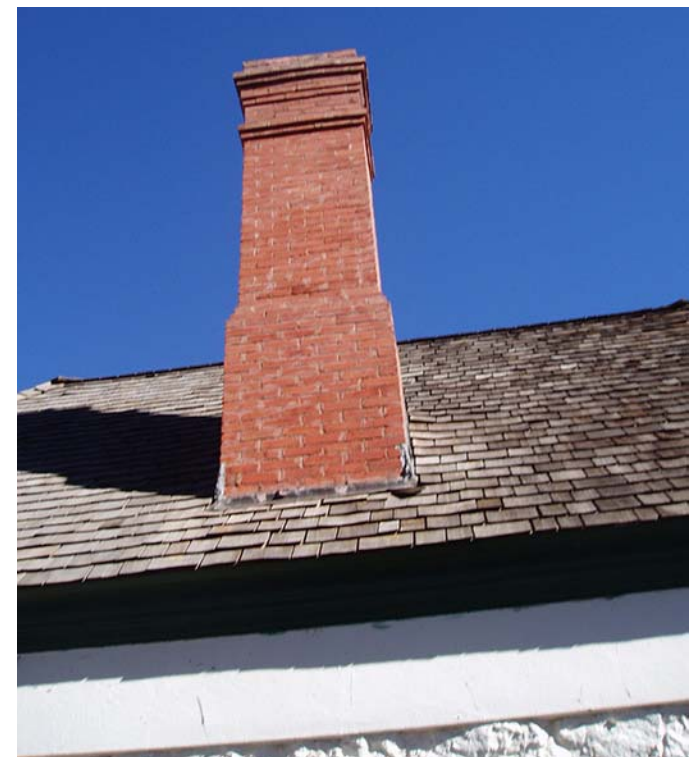
Figure 02 01-13 Chimney at Ft. Stanton, NM.
