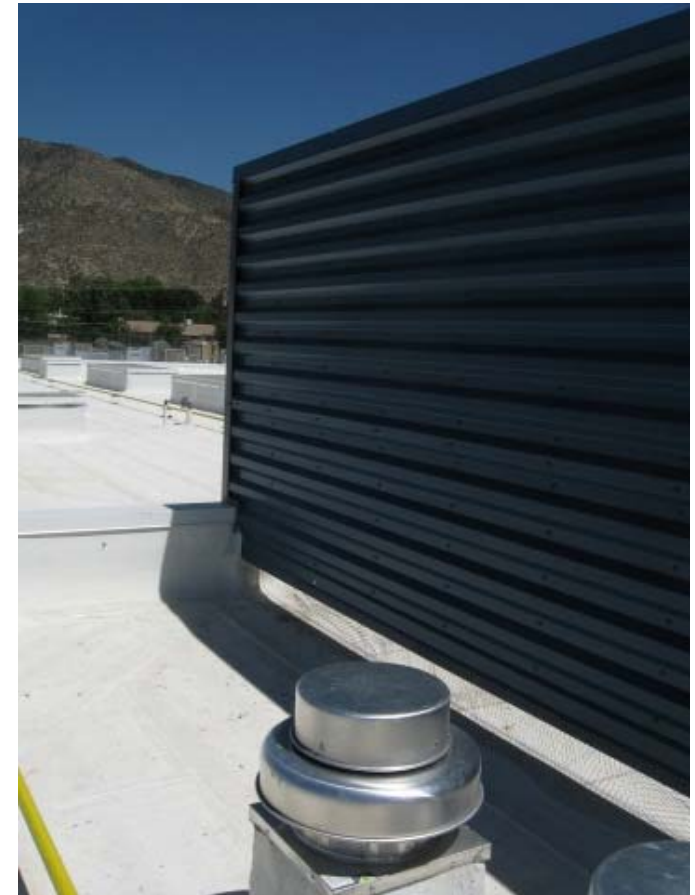
Figure 23 12-1 Rooftop Screen Wall, screens can make the installation of both roof mounted and pad mounted HVAC equipment more acceptable for historic buildings.
