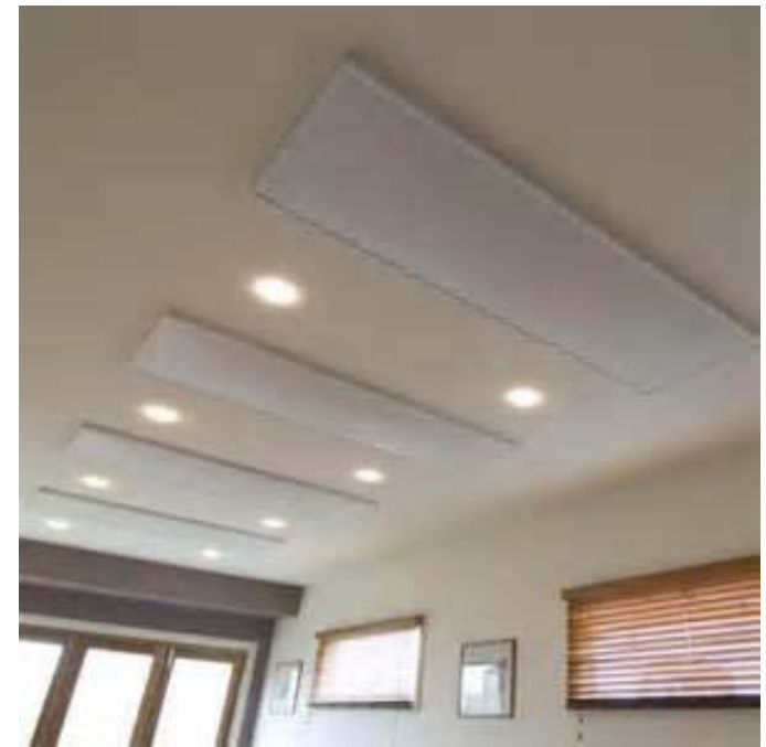
Figure 26 22-2 Picture of ceiling mounted electric radiant heating panels.
