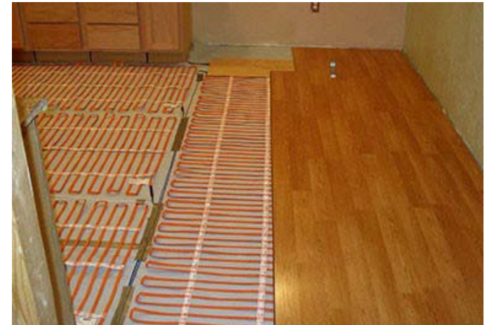
Figure 23 40-4 Electric heating mats being installed under a wood floor system.
