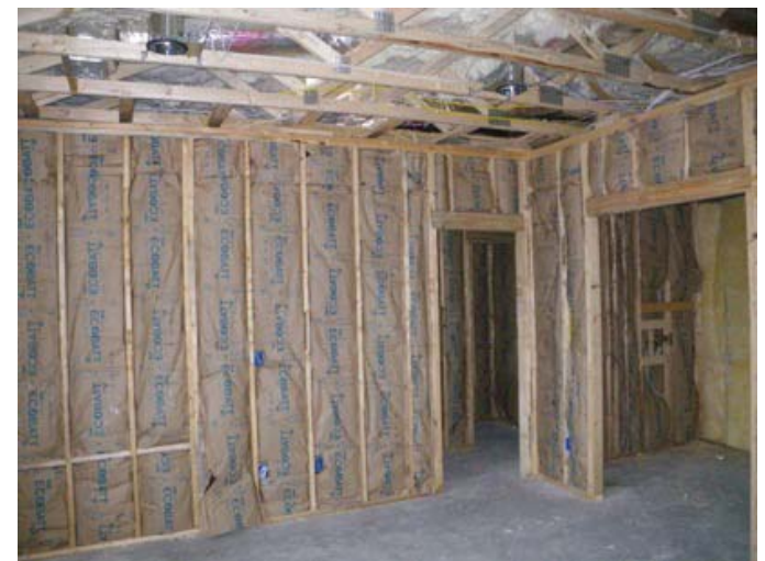
Figure 06 81-10 Installed faced batts in a wood stud wall.
