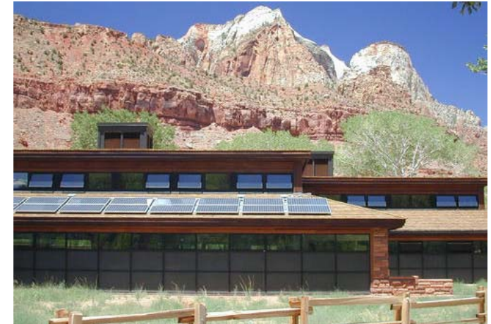
Figure 04 41-6 Photograph of South Façade
