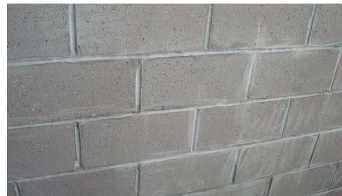
Figure 04 21-1 CMU Wall, above
