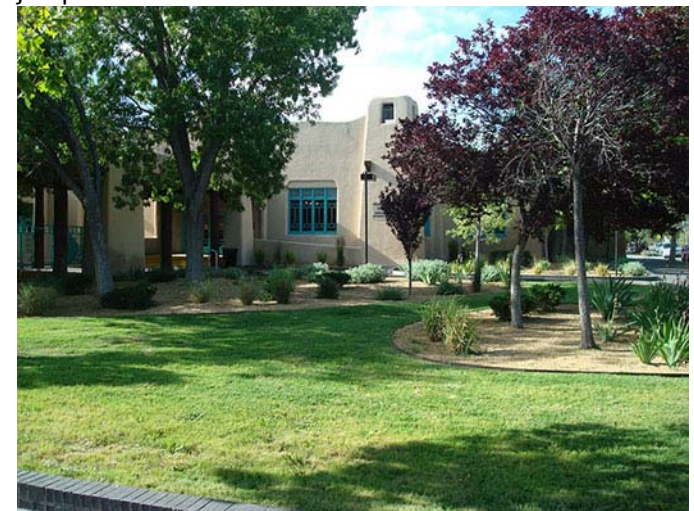
Figure 32 17-11 After: Special Collections Library, Albuquerque, NM. Renovated landscaping maintained the historic character by providing a lawn of desert grass near the pedestrian walks, but added in large areas filled with crusher fines. Juniper shrubs were changed out for other xeric plants and shrubs.
