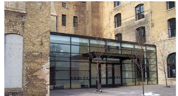
Figure 04 41-7 Note: An example of an acceptable addition to a historic building that can also be a trombe wall. According to Preservation Brief 14 “This glass addition was erected at the back of an 1895 former brewery during rehabilitation to provide another entrance. The addition is compatible with the plain character of the secondary elevation.” (Grimmer et al. 2010).
