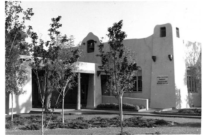
Figure 32 17-10 Before: Special Collections Library, Albuquerque, NM. Historic landscaping consisted of large areas of blue grass ornamented with sections of juniper shrubs.
