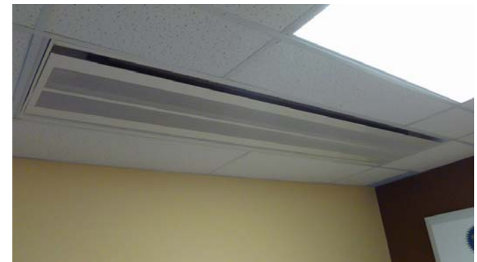
Figure 23 11-4 Contemporary chilled beam
