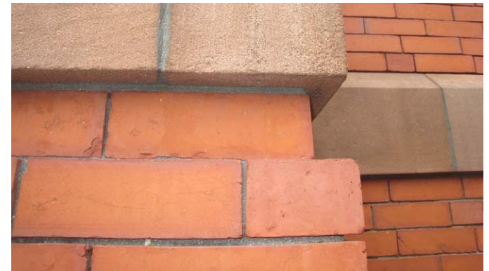
Figure 04 41-2 Repointed Historic brick wall
