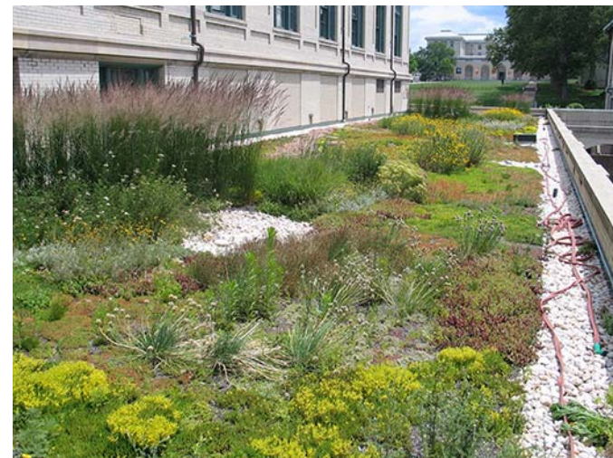
Figure 07 52-4 Semi-Intensive Green Roof
