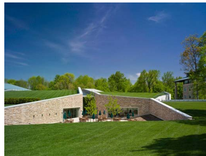
Figure 32 29-9 Earth berm at the Becton Dickinson Campus Center, Franklin Lakes, NJ.
