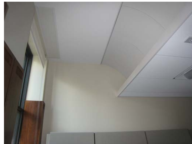
Figure 23 11-15 Ductwork concealed in a new dropped ceiling space, but detailed to respect the historic windows.
