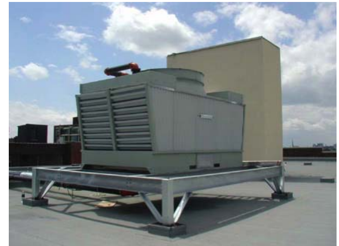
Figure 23 12-7 Cooling Tower
