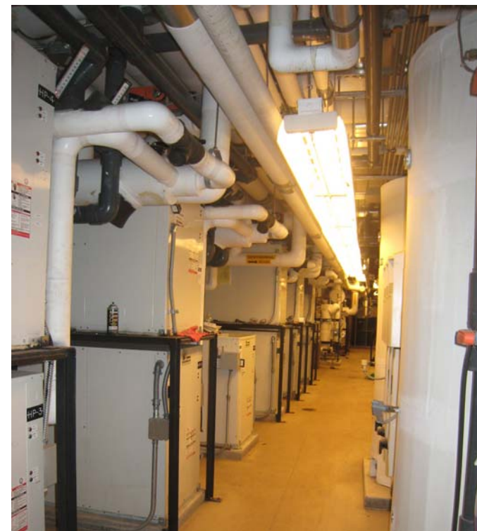
Figure 23 08-16 Heat pumps and blowers at Trinity Church
