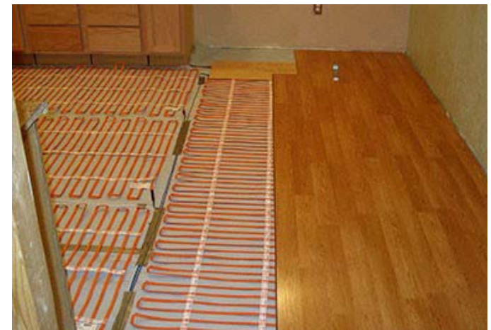
Figure 26 22-5 Electric heating mats being installed under a wood floor system
