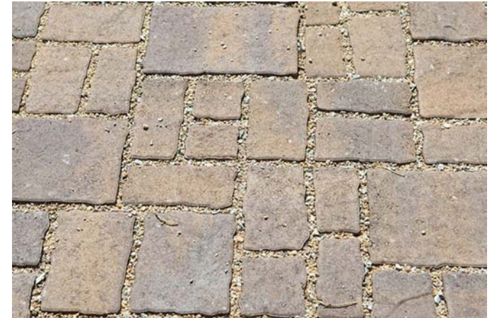
Figure 32 17-4 Permeable Pavers, crusher fines fill joints.
