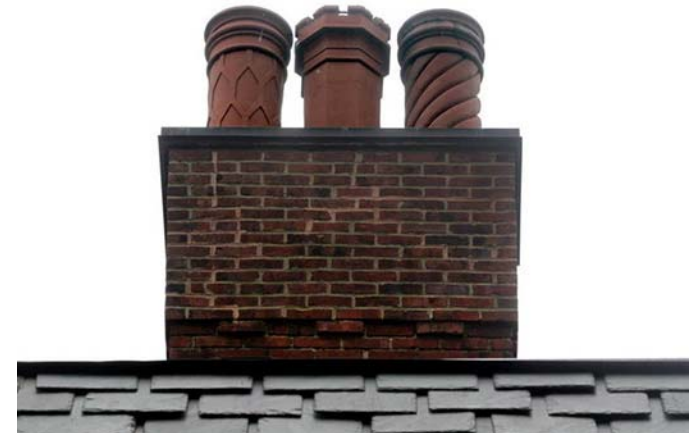
Figure 02 01-12 Historic chimney caps.
