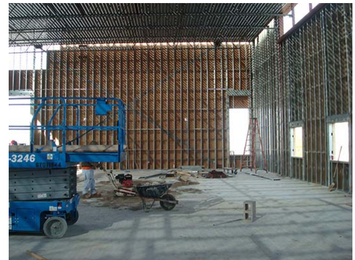
Figure 05 51-8 Metal stud wall, almost ready for insulation.
