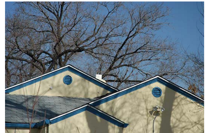
Figure 02 01-19 Attic louvers, Silver Hills Neighborhood, Albuquerque, NM.
