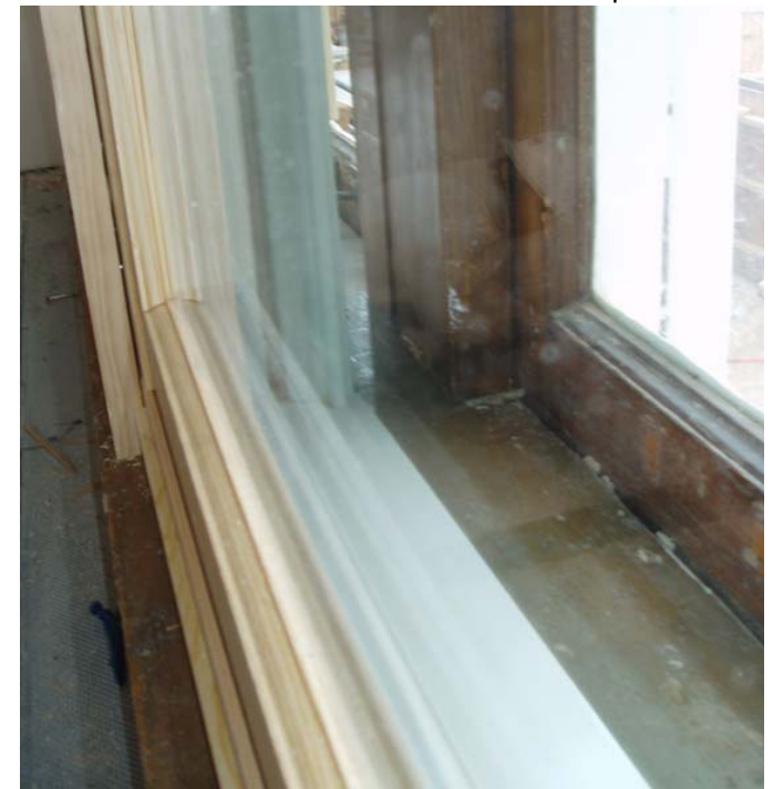
Figure 08 52-3 Close-up of installed interior back-up window
