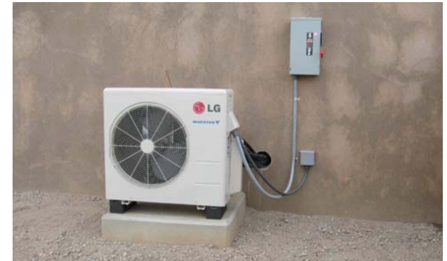
Figure 23 08-11 Pad Mounted Ductless Split Condensing Unit
