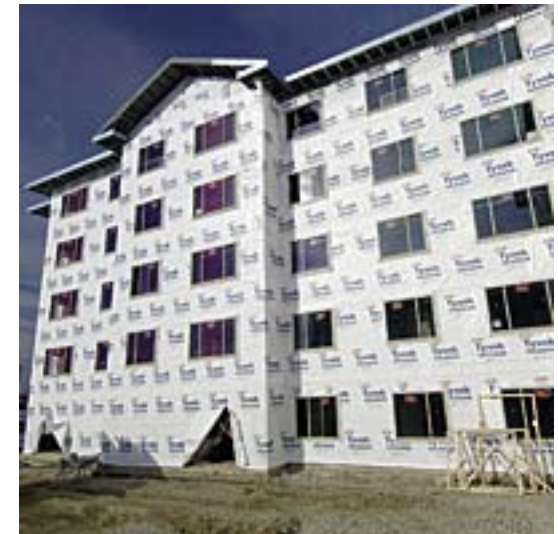
Figure 04 21-8 Sheet barrier, looks like opaque plastic
