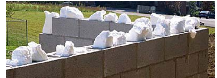
SPRAY FOAM INSULATION ADDED WITHIN MASONRY CAVITY
