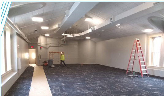
Fort Riley Museum Complex Renovations . Source: U.S. Army
