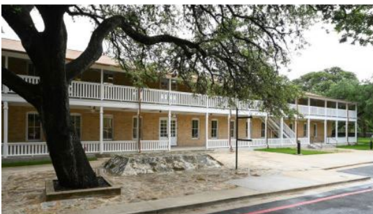
Restored Building 1 at Camp Mabry. Source: 2022 Secretary of Defense Environmental Awards
