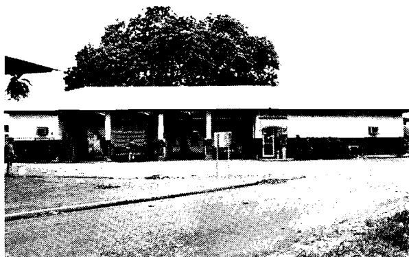
Service Station (Building #53)
