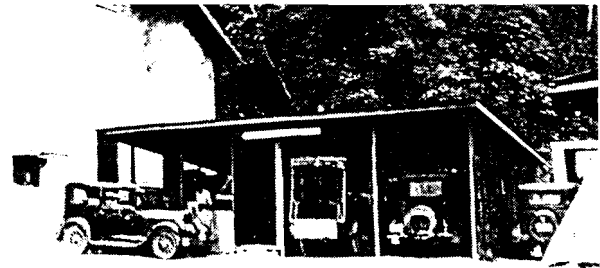
Gas Station - Naos Island
