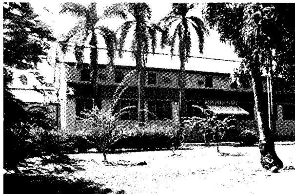
Storehouse building (Building #33)
