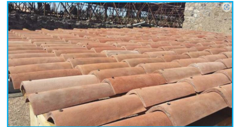
Disguised solar panels as ancient Roman tiles in Pompeii. Source: POCITYF
