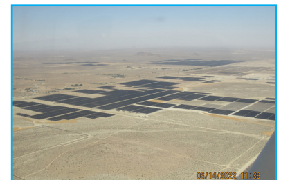
Edwards Solar Array viewed from the air, with construction nearing completion. Source: 412 Test Wing, Edwards AFB.
