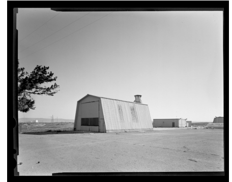
Building on Vandenberg Space Force Base. Source: Photo by Matthew Punke, 2023
