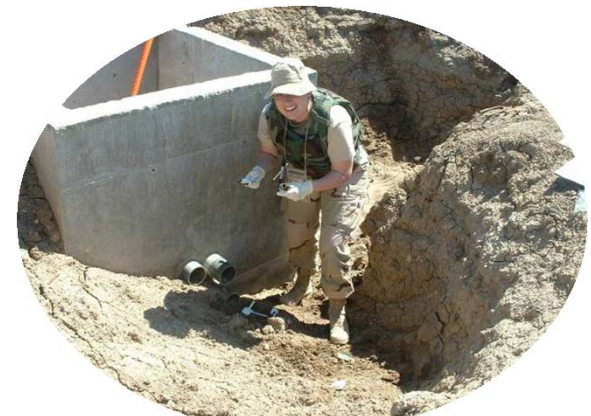
Soil Sampling at Com Manhole
