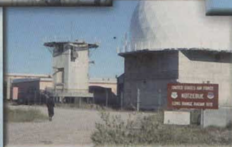
Kotzebue Long Range Radar Site, Kotzebue, AK Photos by Chris Eberly.
