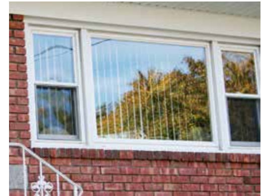
Reflections on home windows are a significant source of bird mortality. The partially opened vertical blinds here may break up the reflection enough to reduce the hazard to birds. Photo by Christine Sheppard, ABC
