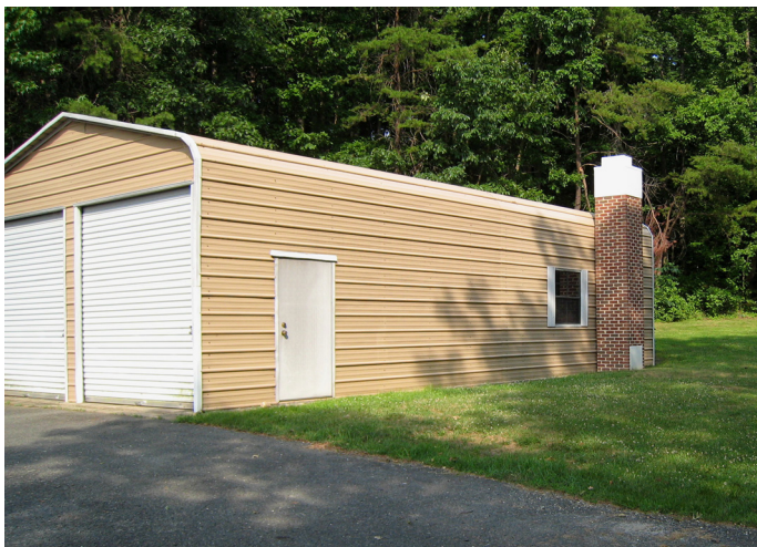
The chimney structure in this photo is the replacement Chimney Swift tower that was erected and utilized during spring 2010 migration.
