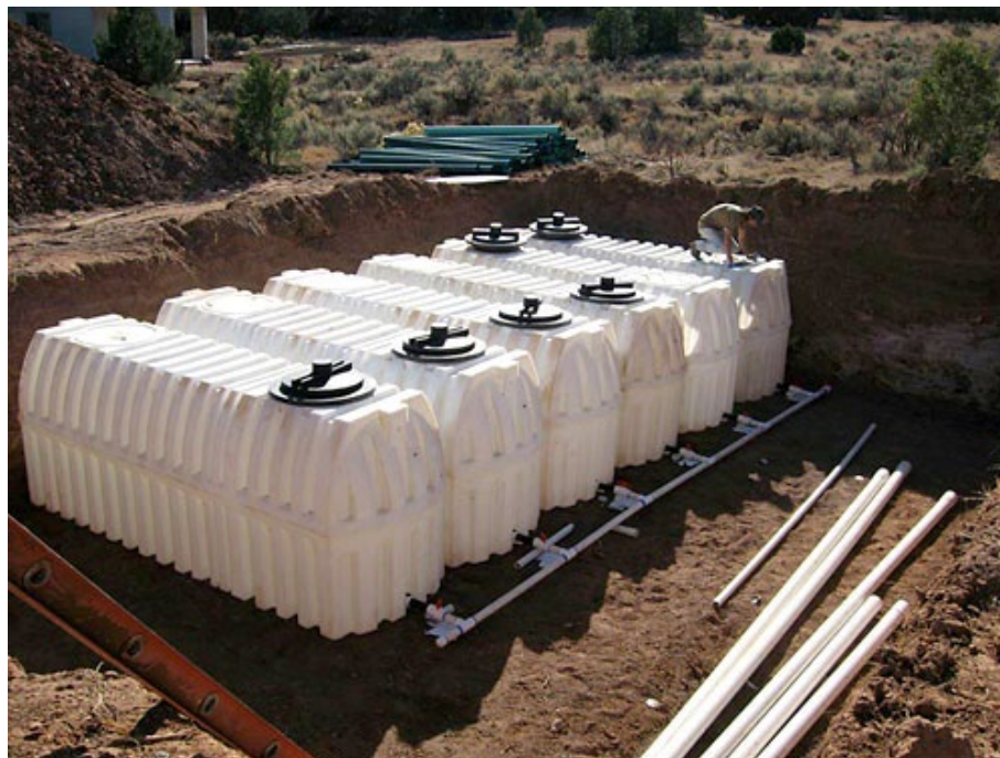
Figure 9. Installation of a large underground cistern system (www.theraincatcherinc.com).
