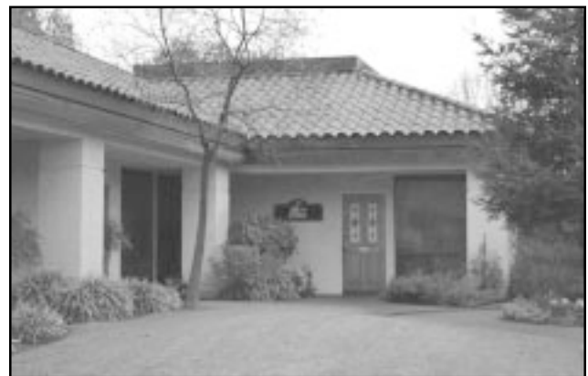
Figure 28. Applied Earthworks is located in a stucco building.
