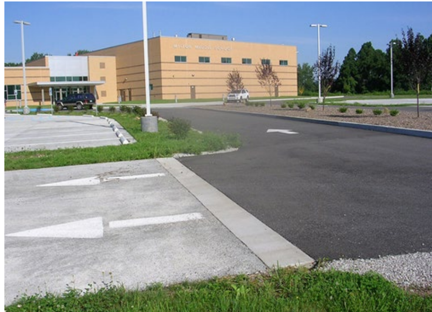
Figure 8. Permeable concrete used throughout a parking lot (www.dep.wv.gov).
