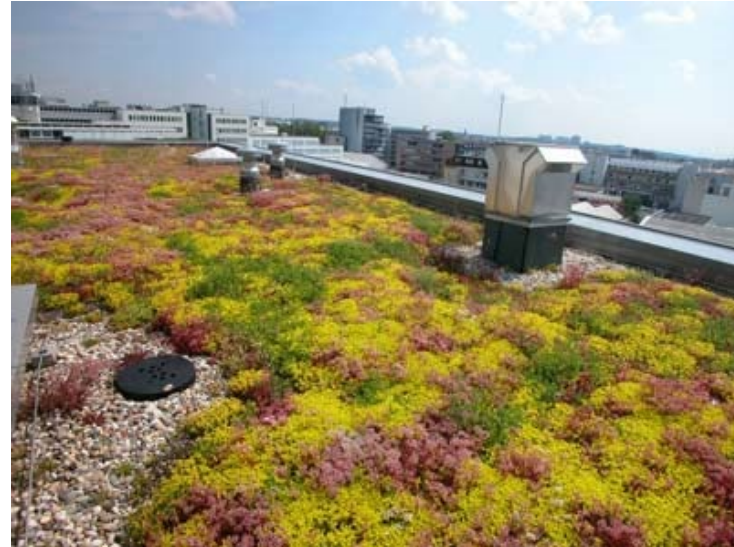
Figure 12. A developed extensive green roof system that has a low profile ( www.enviromat.co.uk ).
