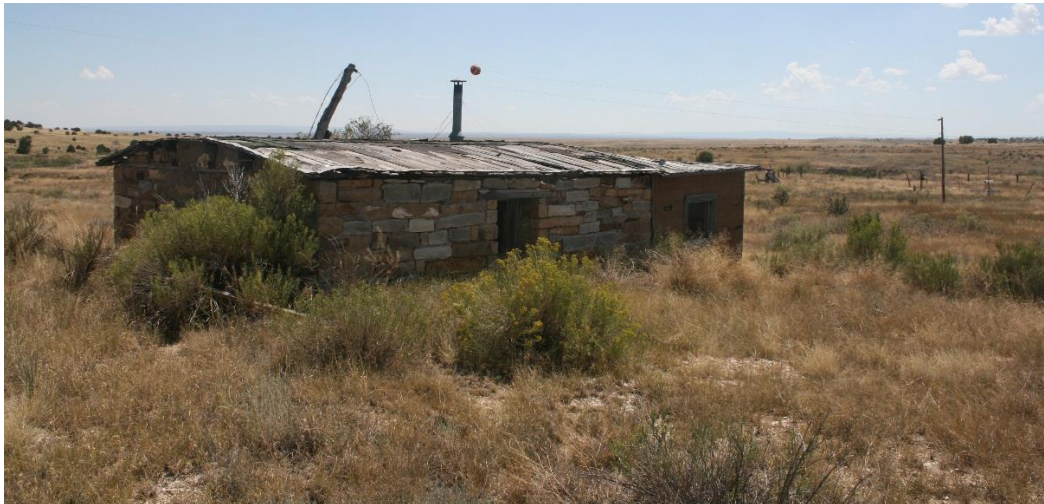
Figure 100. 5LA5820 Feature 7. View from NE to SW.
