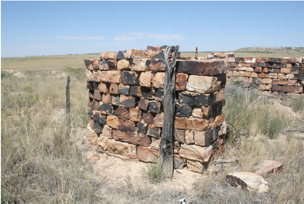
Figure 96. 5LA4406 Feature 3 showing opening, posts and wire fencing. View from E to W.
