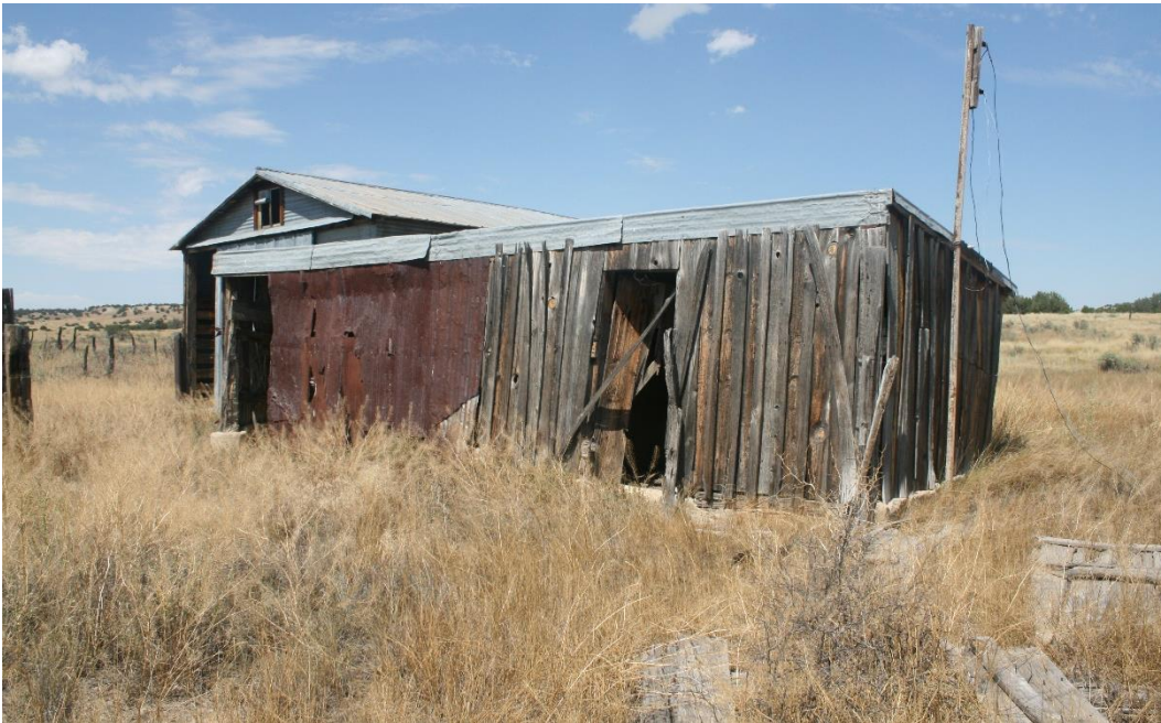
Figure 101. 5LA5820 Feature 2. View from SE to NW.
