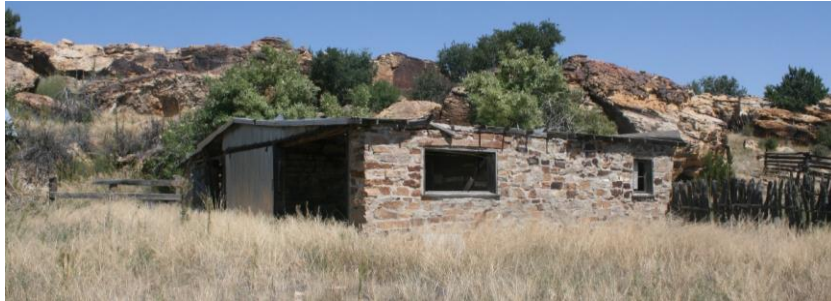
Figure 106. 5LA5830 Feature 3. View from SW to NE.
