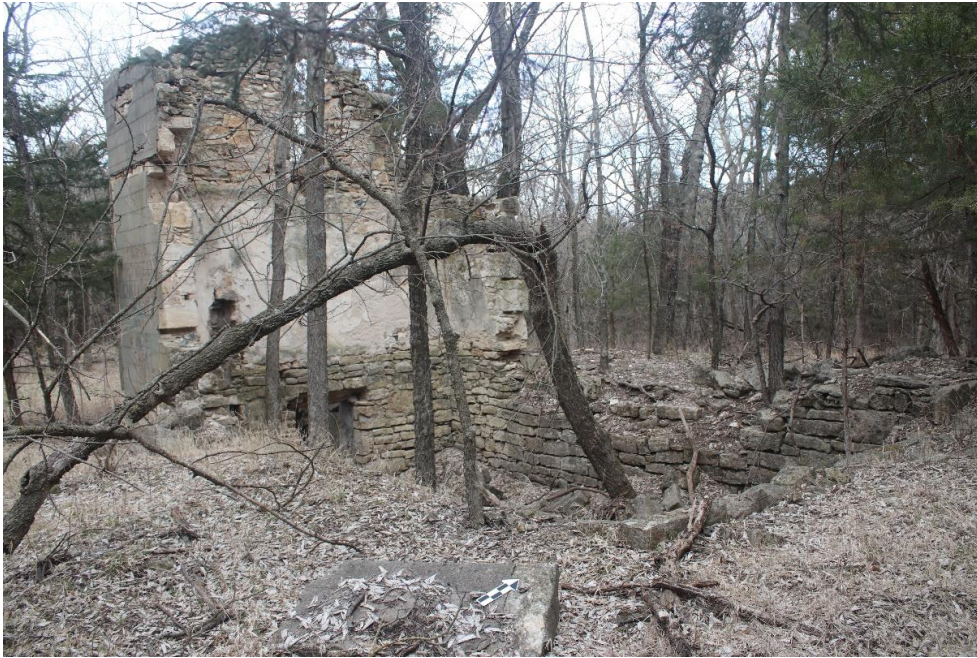
Figure 31. 14RY2140 Feature 9. View from SE to NW.
