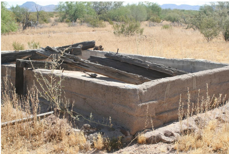
Figure 65. Site AZ Z:5:10 Feature 5 and 6. View from SW towards NE.
