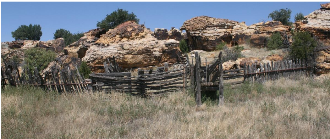
Figure 105. 5LA5830 Feature 2. View from S to N.
