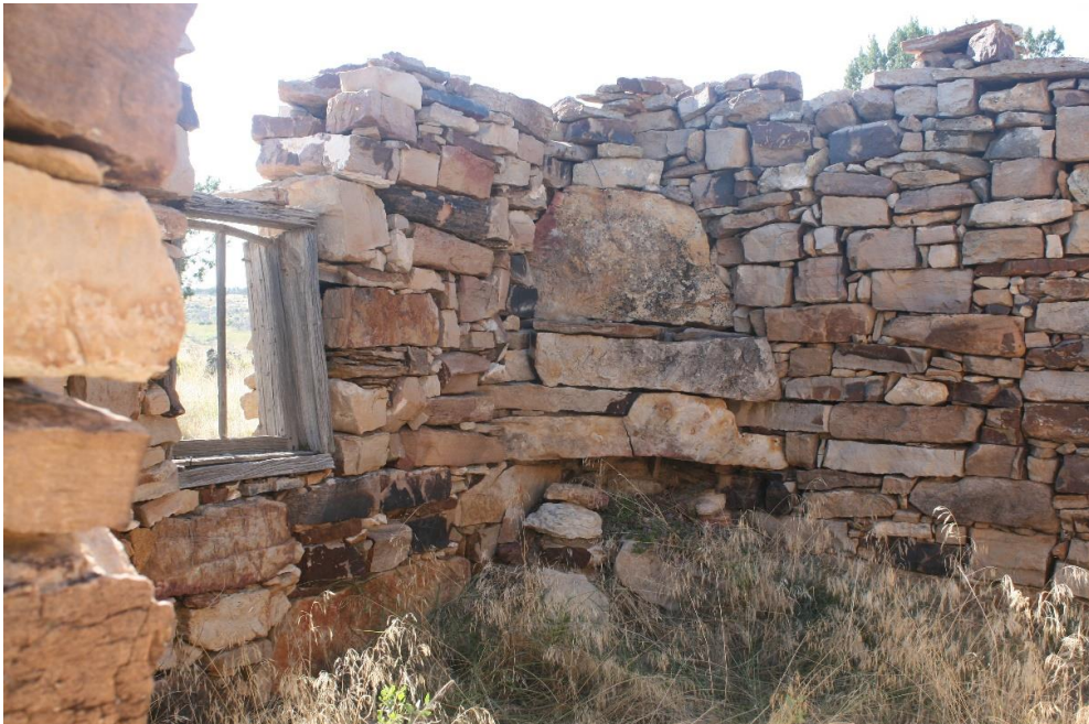
Figure 112. 5LA6140 Feature 4 interior. View from N to S.
