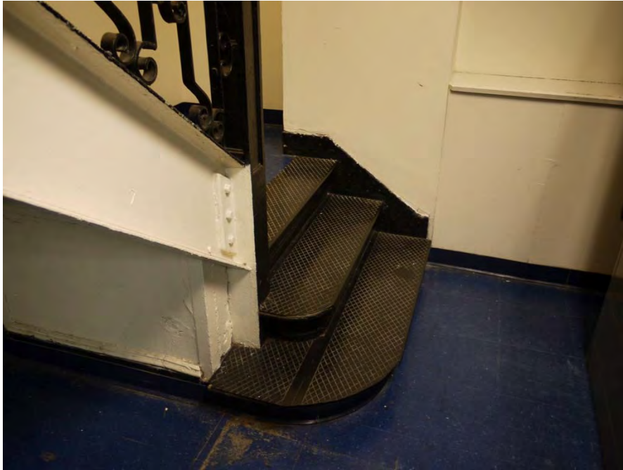
Figure 6.5: Building 8 second floor staircase.
