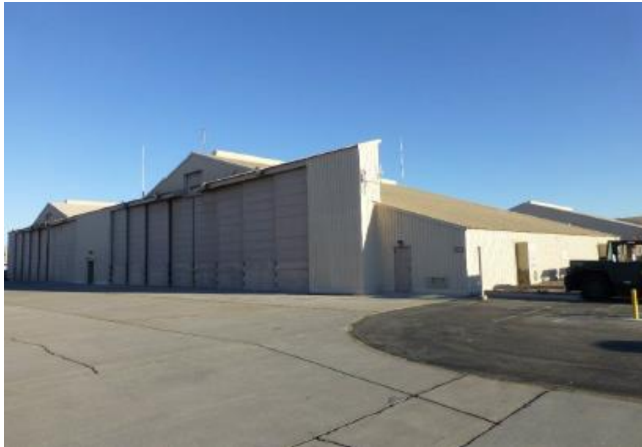
Building 222: Red Flag Maintenance Hangar
