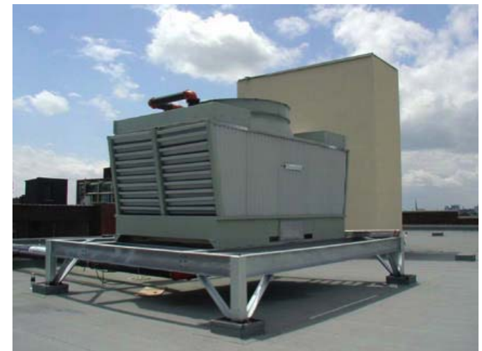
Figure 23 12-7 Cooling Tower
