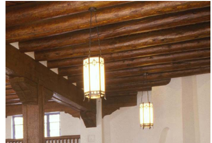
Figure 26 51-3 Old Terminal, Albuquerque, New Mexico The historic fixtures were found in local museum but were not reinstalled because obtaining the UL rating was time consuming and prohibitively expensive. Therefore, the historic fixtures were replicated and can be seen in the above photograph.
