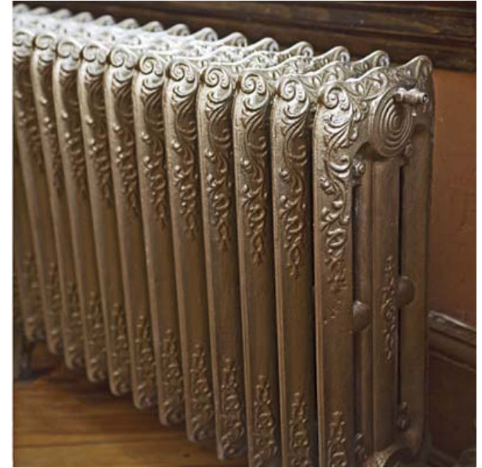
Figure 23 08-18 Historic steam radiator for a Two-Pipe Radiant Heating system. Not only can the radiator be reused, but it also might be considered a character-defining feature. If steam radiators are present in the building being renovated, discuss option with the Design Team and CRM/SHPO.
