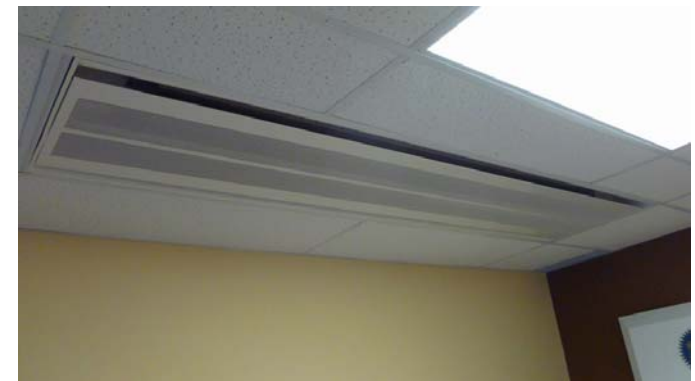
Figure 23 11-4 Contemporary chilled beam
