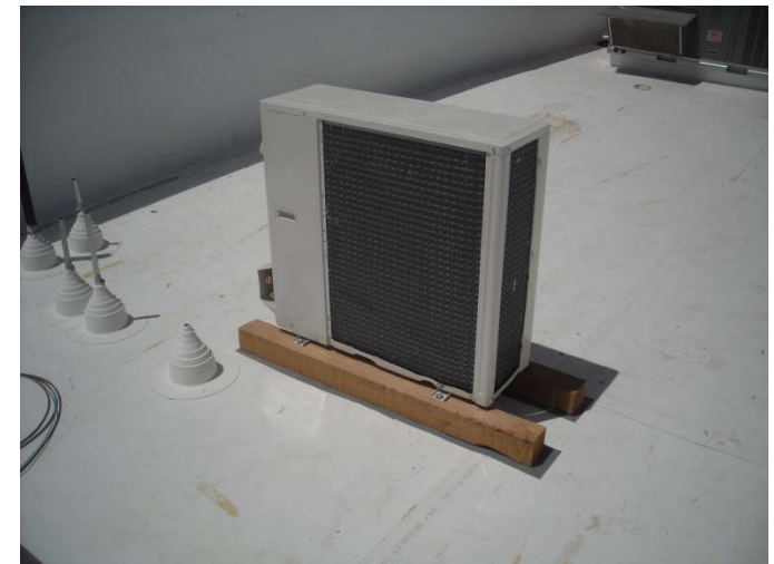
Figure 23 12-9 Roof Mounted Condensing Unit for ductless split system
