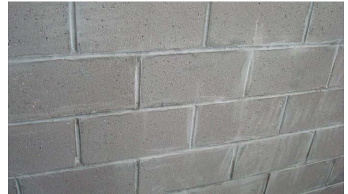
Figure 04 21-1 CMU Wall, above
