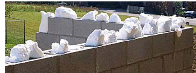
SPRAY FOAM INSULATION ADDED WITHIN MASONRY CAVITY
