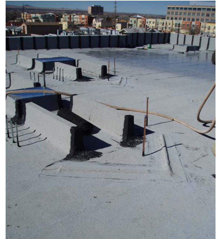
Figure 07 51-1 New insulation and built-up roof applied to historic Coronado School, Albuquerque, New Mexico.
