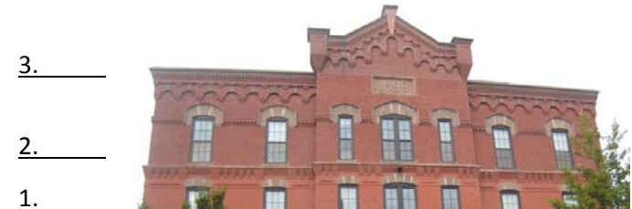
Figure 07 01-1 Numbers reflect different additions and renovations that can be seen in the cornice detailing and brick color.
