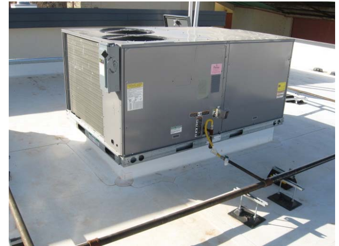
Figure 23 12-4 Packaged Rooftop Unit with Gas Heat
