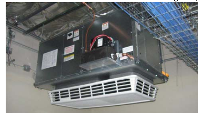
Figure 23 08-13 Interior Split-System Evaporator Coil, For Figures 23 08-11 & 12, see diagram on page 110 for component locations.
