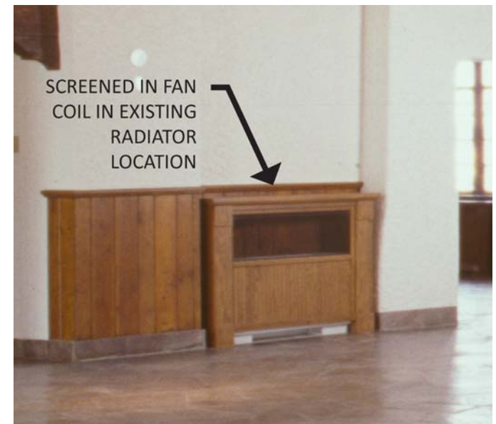
Figure 23 08-10 Old Terminal Building, Albuquerque International Sunport, New Mexico
