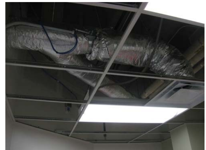
Figure 23 11-16 Insulated ductwork installed above new lay-in ceiling (ceiling tiles not installed yet)
