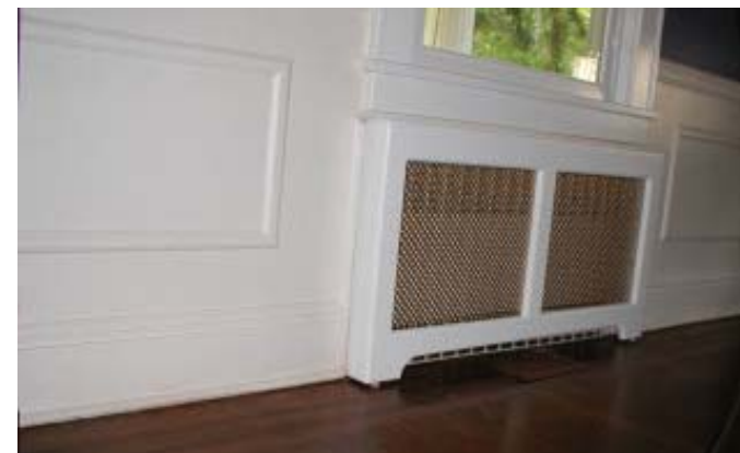
Figure 23 11-6 Radiator furred into the wall
