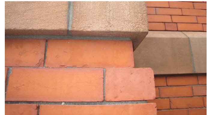
Figure 04 21-2 Repointed Historic brick wall, above
