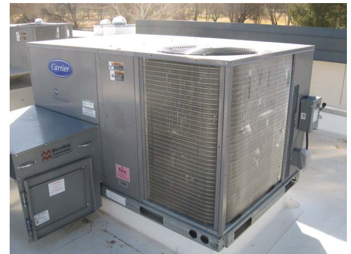
Figure 23 12-3 Packaged Rooftop Unit with Economizer
