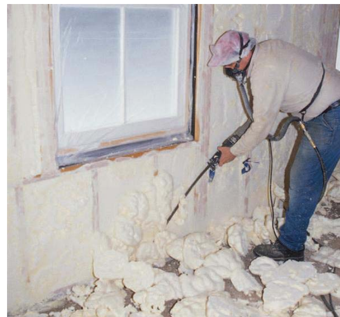
Figure 06 81-11 Trimming is not a feasible option in an Historic Structure
