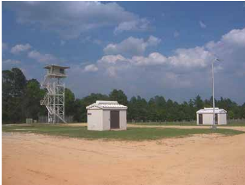
Figure 519. Control tower and range buildings, Fort Bragg, NC, 17 May 2006.
