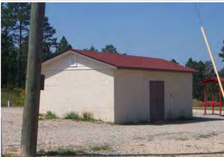
Figure 531. Range storage building, Fort Bragg, NC, 17 May 2006.
