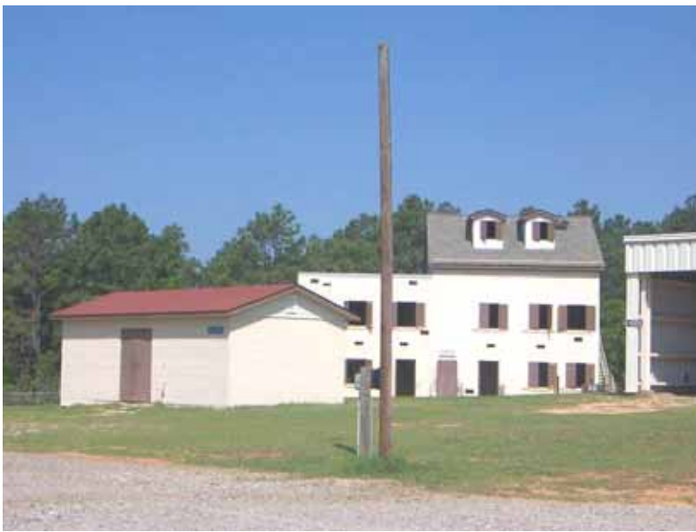
Figure 533. Range storage building, Fort Bragg, NC, 17 May 2006.
