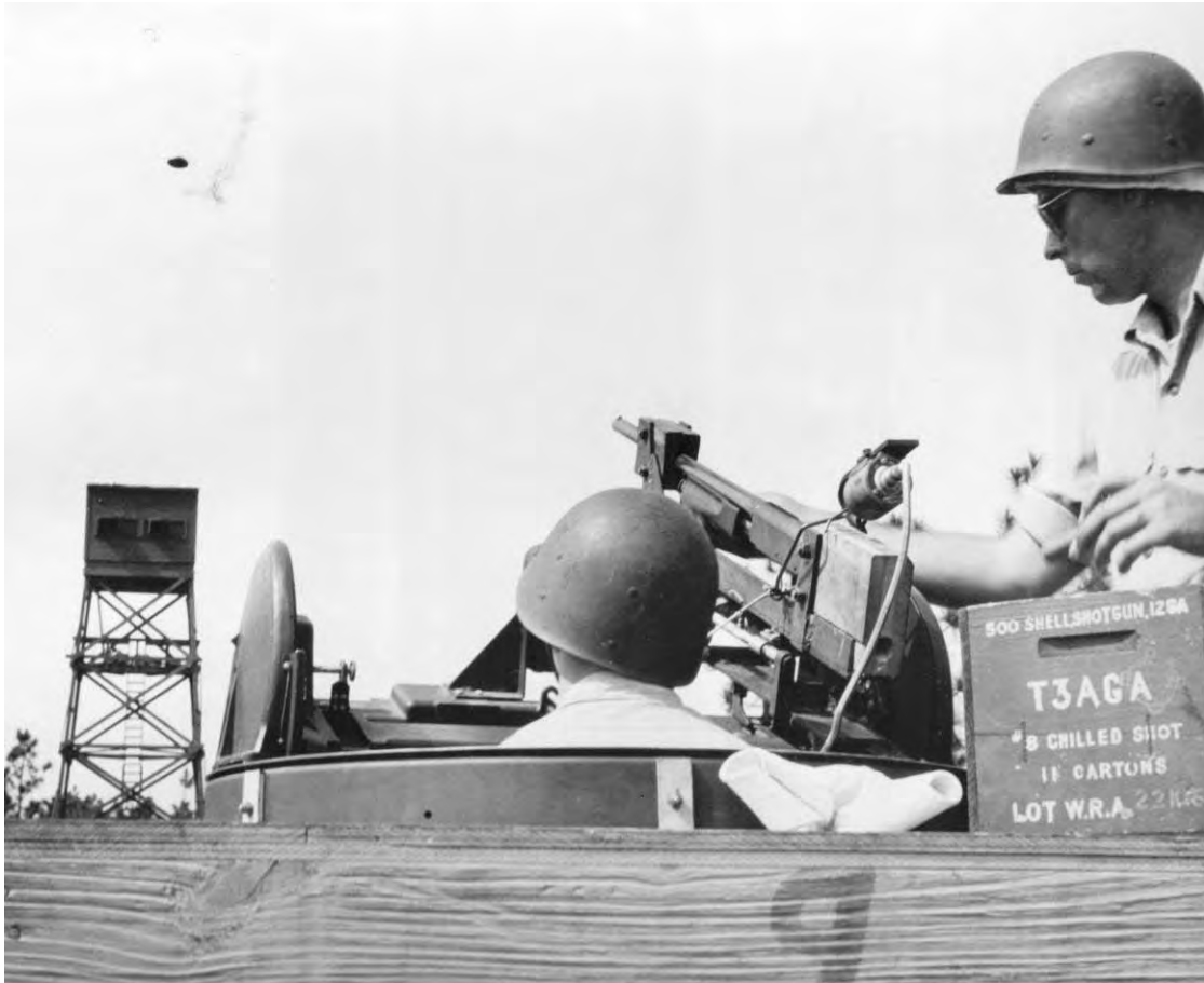
Figure 53. High tower and turret range NAGS shot gun range at NAS Jacksonville, FL, 27 February 1944 (NARA College Park, RG 80-G, box 740, photo 241829).
