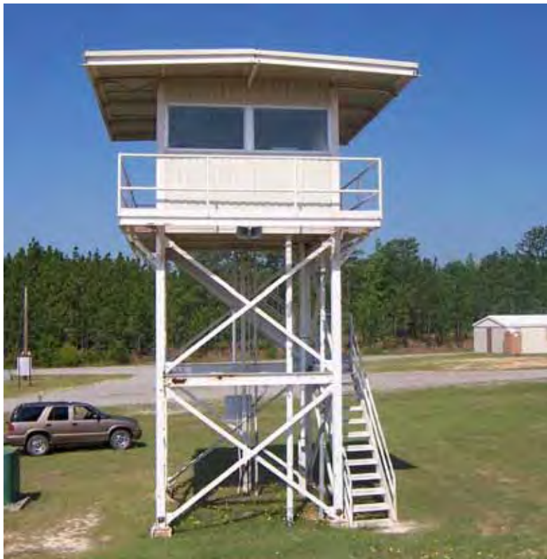
Figure 520. Observation tower, Fort Bragg, NC, 17 May 2006.
