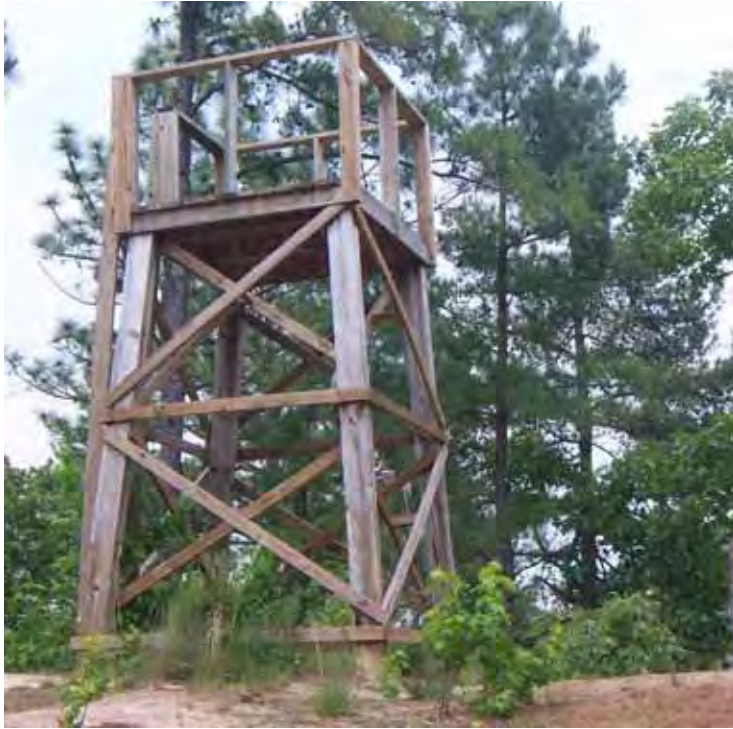
Figure 514. Observation tower, Fort Bragg, NC, 17 May 2006.
