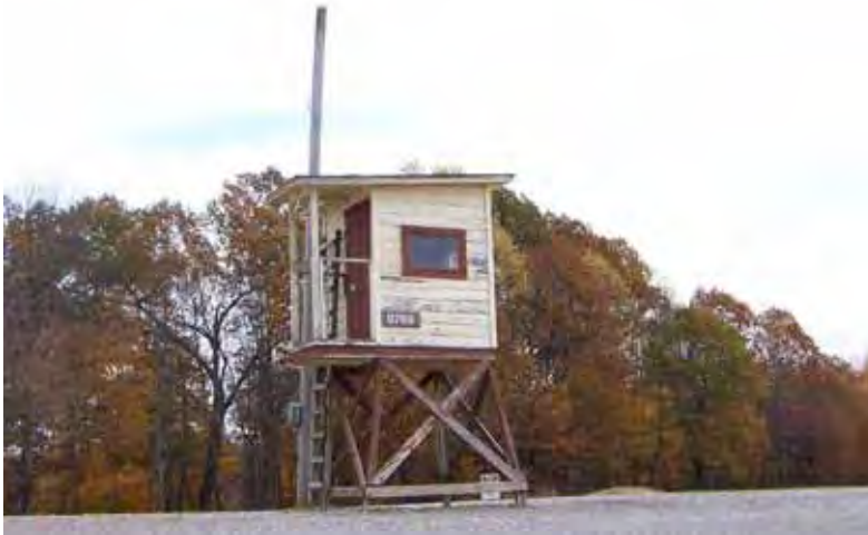
Figure 510. WWII Observation Tower Building 9789, Fort Knox, KY, November 2005.
