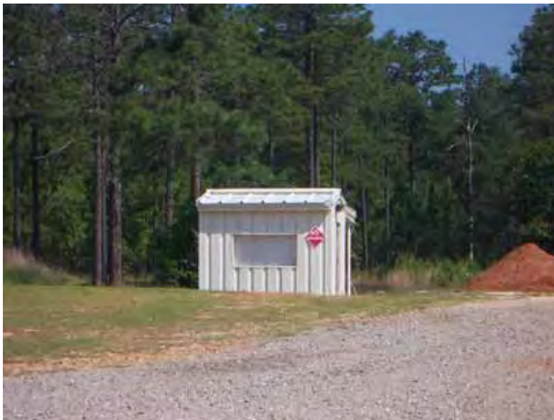
Figure 534. Range storage building, Fort Bragg, NC, 17 May 2006.
