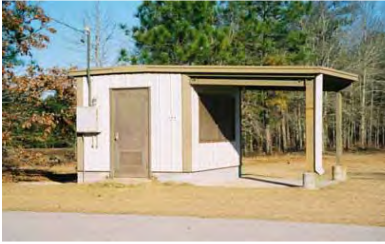
Figure 535. 1987 Building 485 range storage, Fort Gordon, January 2004.
