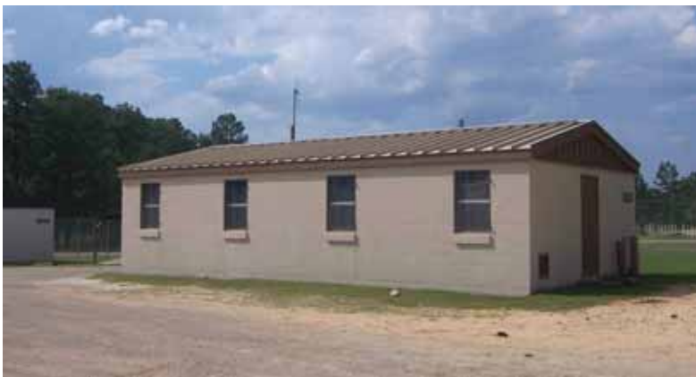
Figure 530. Range storage building, Fort Bragg, NC, 17 May 2006.
