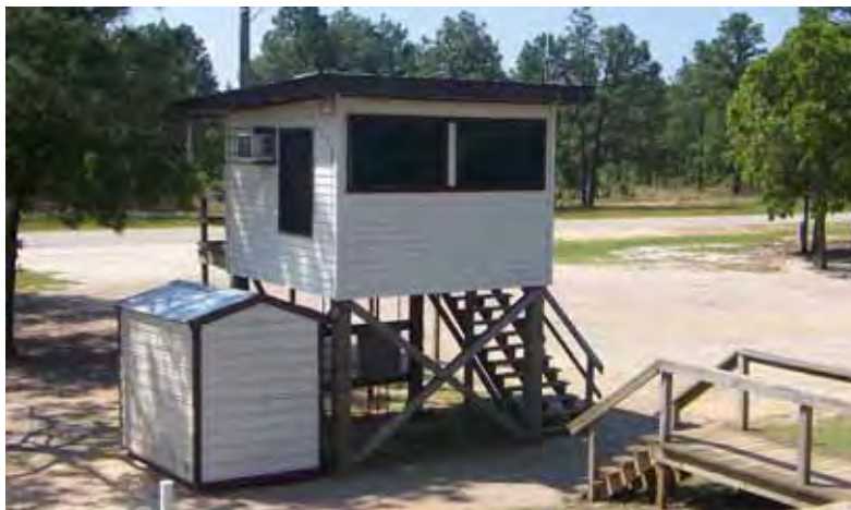
Figure 522. Observation tower, Fort Bragg, NC, 17 May 2006.
