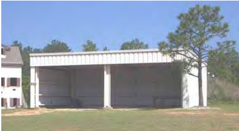
Figure 532. Range storage building, Fort Bragg, NC, 17 May 2006.
