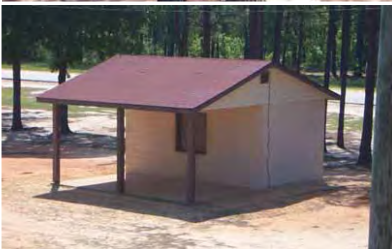
Figure 537. Range ammunition storage building, Fort Bragg, NC, 17 May 2006.
