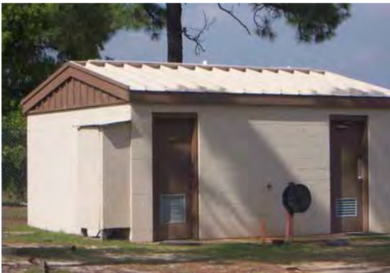
Figure 544. Range latrine, Fort Bragg, NC, 17 May 2006.
