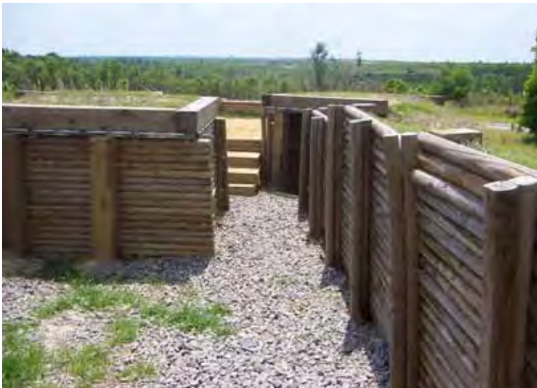
Figure 497. Walled embankments at grenade range firing lines, Fort Bragg, NC, 17 May 2006.
