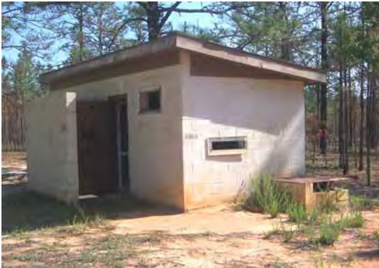
Figure 543. Range latrine, Fort Bragg, NC, 17 May 2006.
