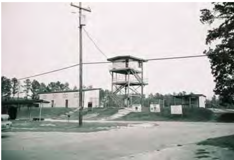
Figure 547. 1995 Range 10 observation tower and grandstand, Fort Jackson, SC, July 2003.
