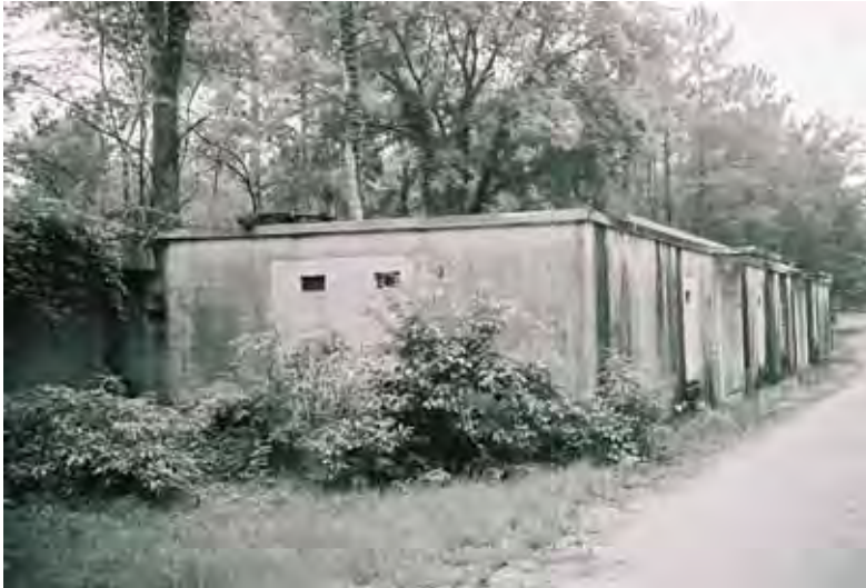
Figure 542. remnants of wwii known distance range target butt, latrine, and target storage, Fort Jackson, SC (SCARNG), June 2004.
