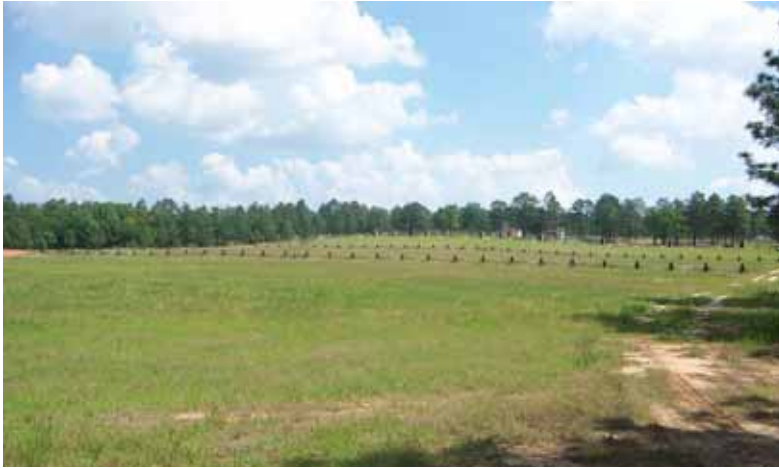
Figure 465. Transition Range, Fort Bragg, NC, 17 May 2006.
