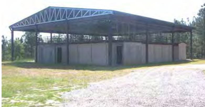
Figure 523. Range firing tower, Fort Bragg, NC, 17 May 2006.
