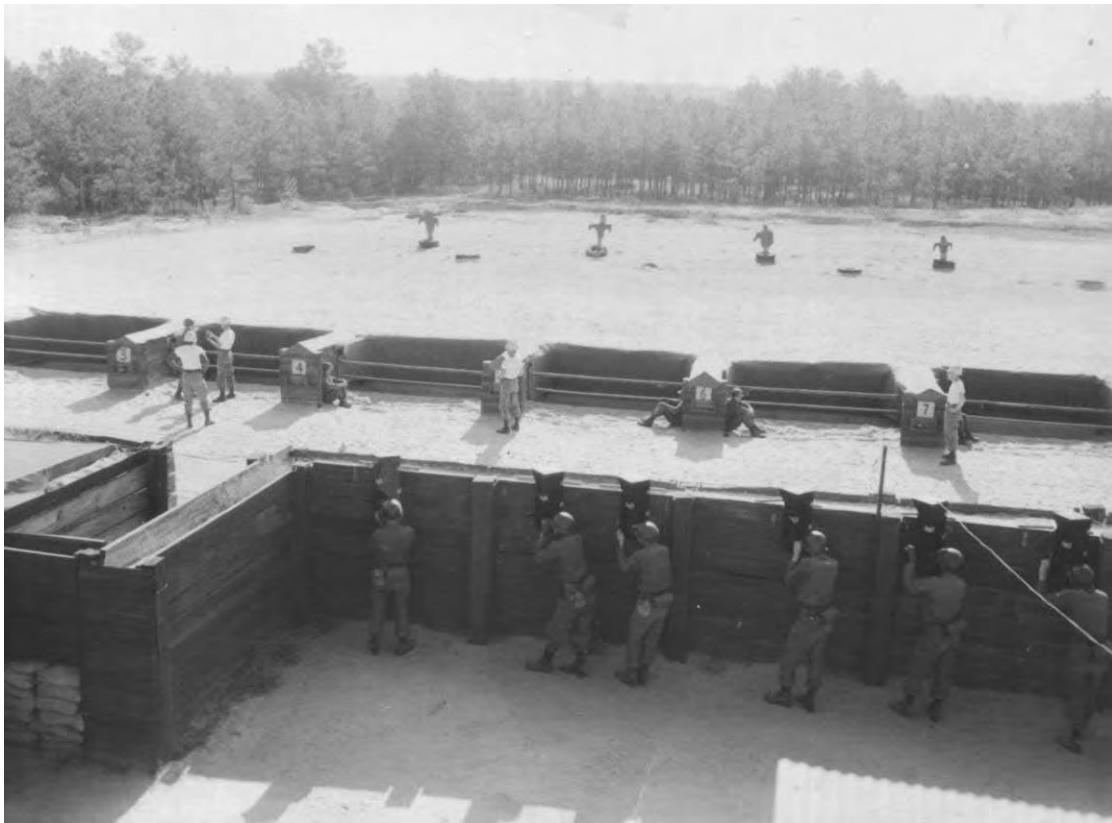
Figure 364. Periscopes, throwing bays, and impact area at Remagen Hand Grenade Range at Fort Jackson, SC, 1 November 1961 (NARA College Park, RG 111-SC post-1955, box 371, photo SC592064).
