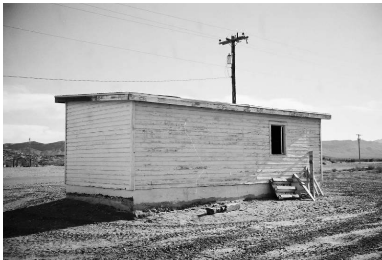
Figure 525. WWII Range Target Storage Bldg 9898, Fort Bliss, TX, November 2005.
