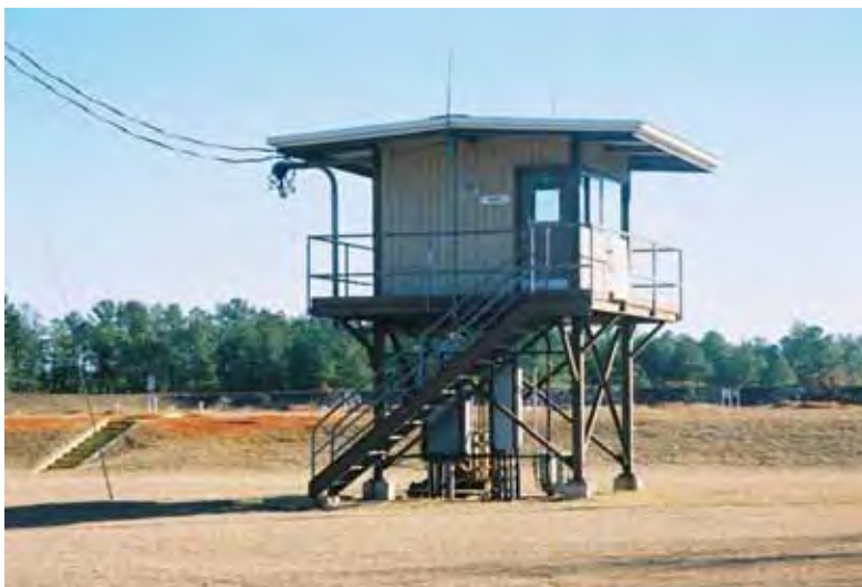
Figure 517. 1987 Range Bldg 486, Fort Gordon, GA, January 2004.
