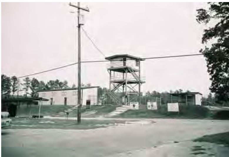
Figure 518. 1995 Range 10 observation tower and grandstand, Fort Jackson, SC, July 2003.
