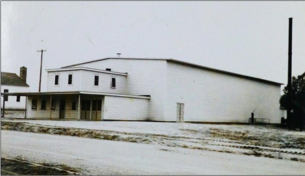
Figure 76. Movie Theater in the segregated portion of the Fort Custer cantonment, 1941 (NARA College Park 77-393-302).
