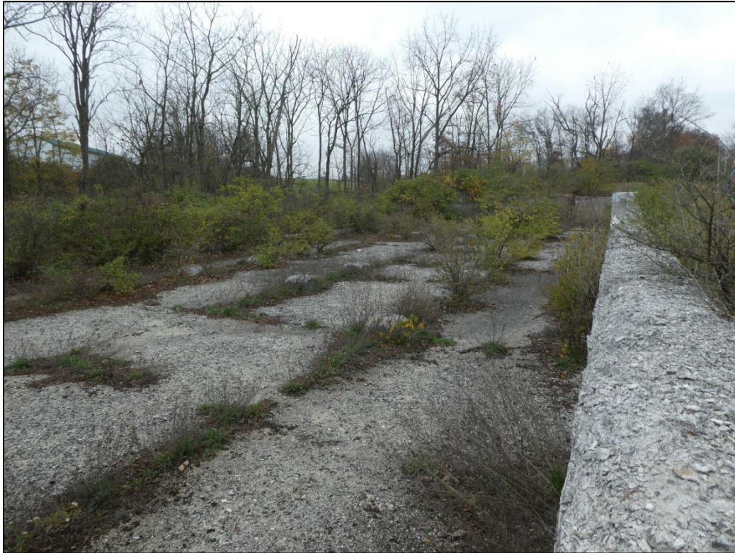
Figure 149. Concrete foundations of dry-land ships, 2020 (ERDC-CERL).
