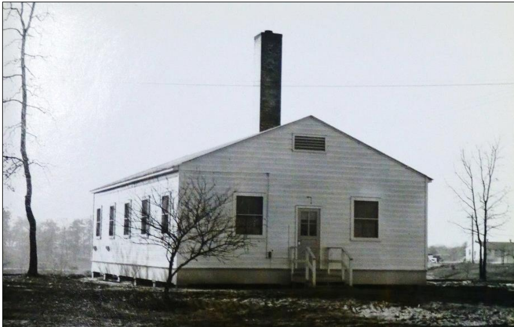
Figure 75. Guest House in the segregated portion of the Fort Custer cantonment, 1941 (NARA College Park 77-393-302).
