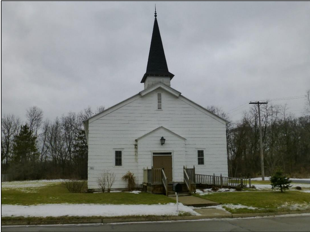
Figure 144. Chapel (Building 651) now in private ownership (ERDC-CERL 2016).
