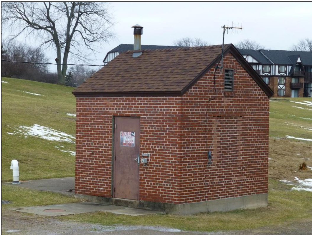
Figure 147. Sewage Pump Station (Building 729) ownership unknown (possibly city of Springfield) (ERDC-CERL 2016).
