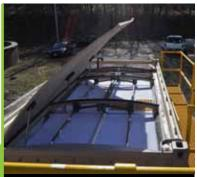
Secondary treatment unit with open access to textile filters
