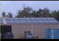
Before the photovoltaic array was installed at Camp Katuu, PACOM and A/249th Engineering Battalion designed and incorporated modifications to reinforce the roof to support the additional weight of the solar panels and mounting equipment, currently estimated to be 10,500 pounds.
