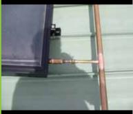
Solar panels attached to existing metal roof with special clips
