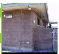
Installed copper under soffit to equipment pad
